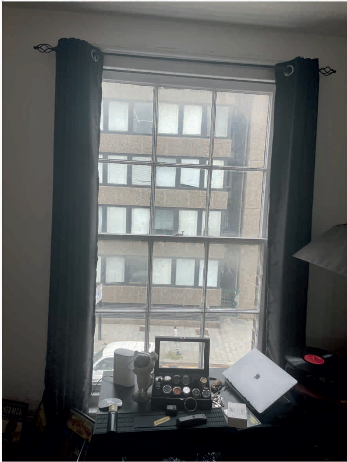
ROOM 22 - Original sash window left hand to be made good and secondary internal glazing installed.
