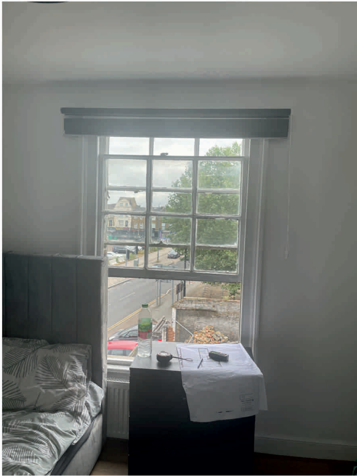
ROOM 21 - Original sash window to be made good and secondary internal glazing installed. Original skirtings remain intact. No cornice.
