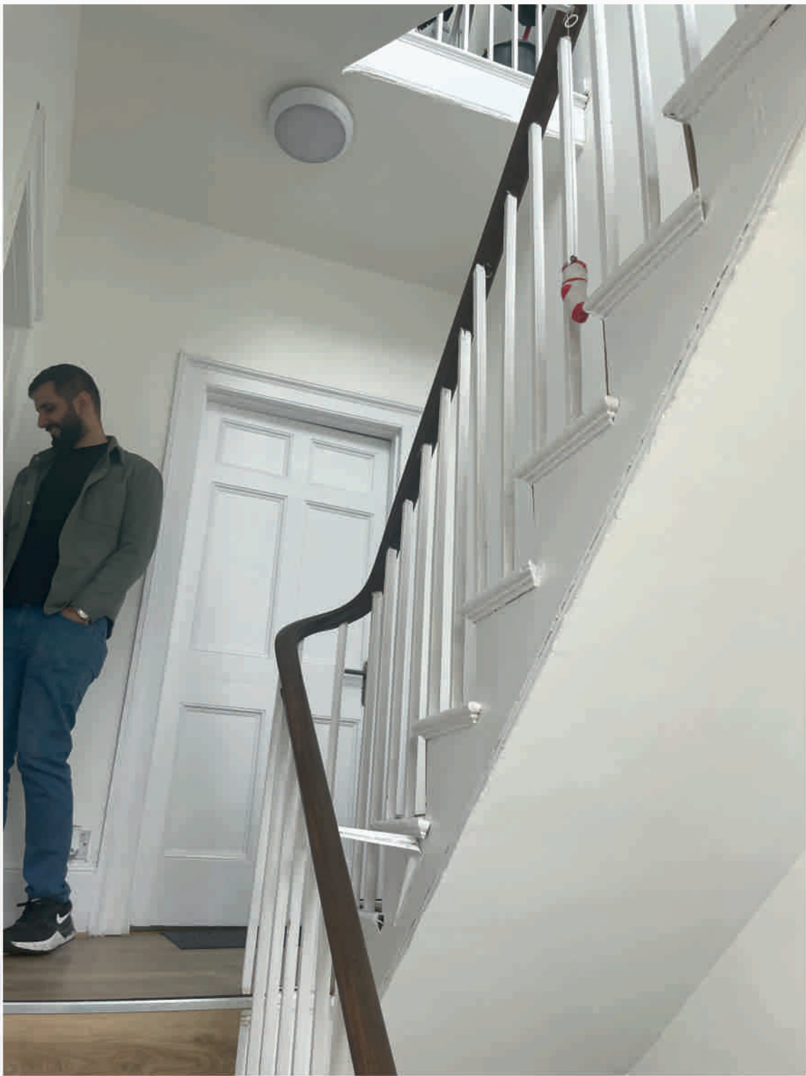
STAIR ENCLOSURE 15 - Showing original stair features to second floor all to remain.
