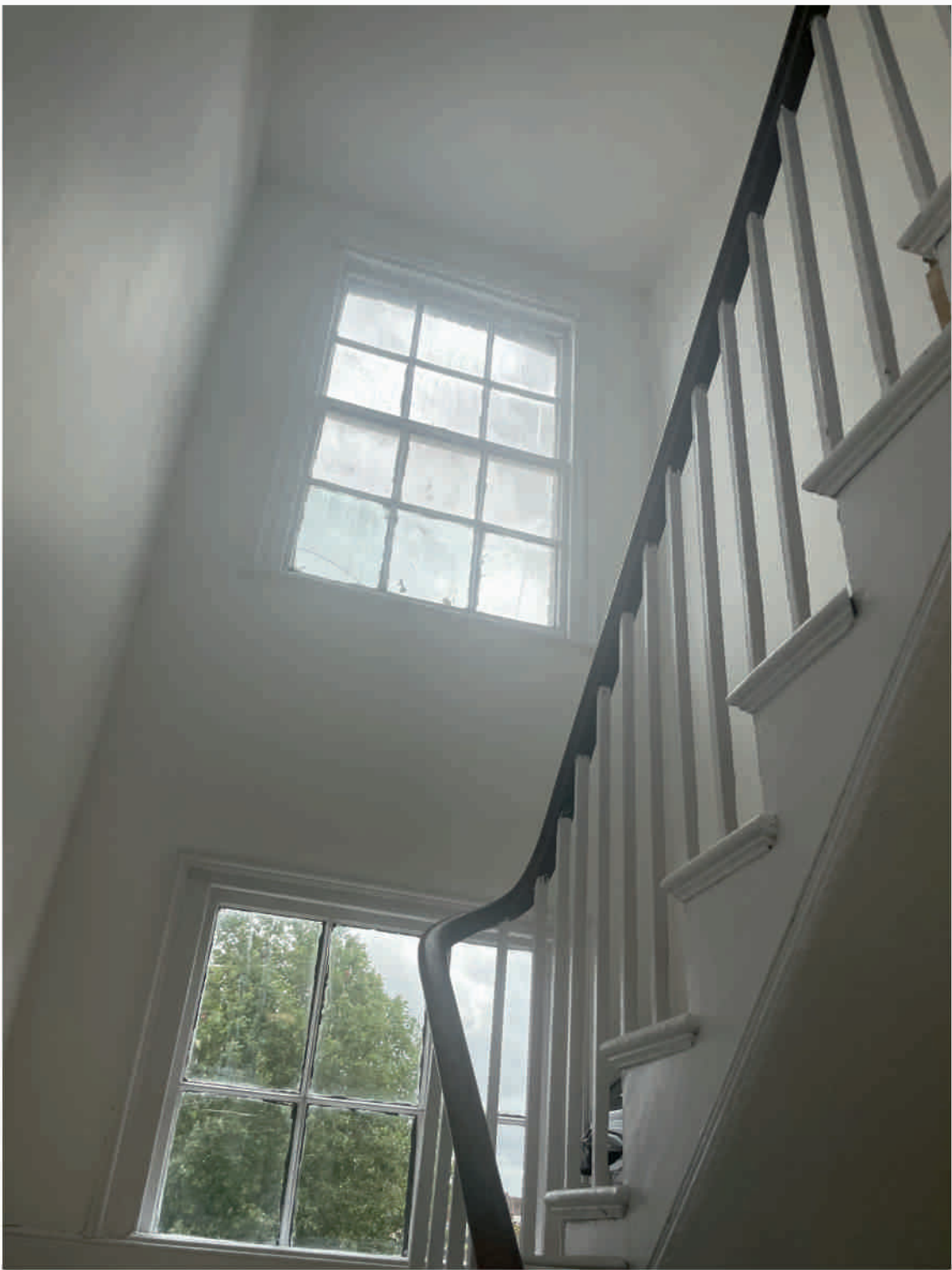
STAIR ENCLOSURE 20 - Showing original to hung window at half landing to second floor. Not original handrail, balusters, cut string and nosings all to remain intact.
