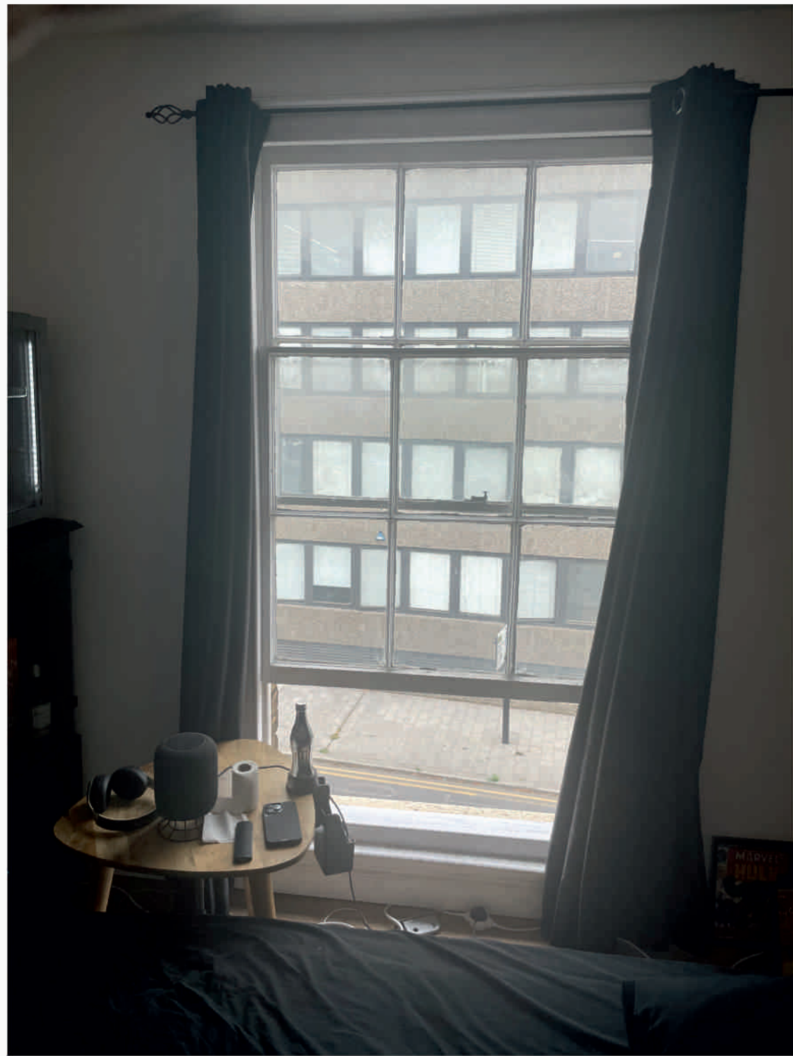
ROOM 22 - Original sash window right hand to be made good and secondary internal glazing installed.
