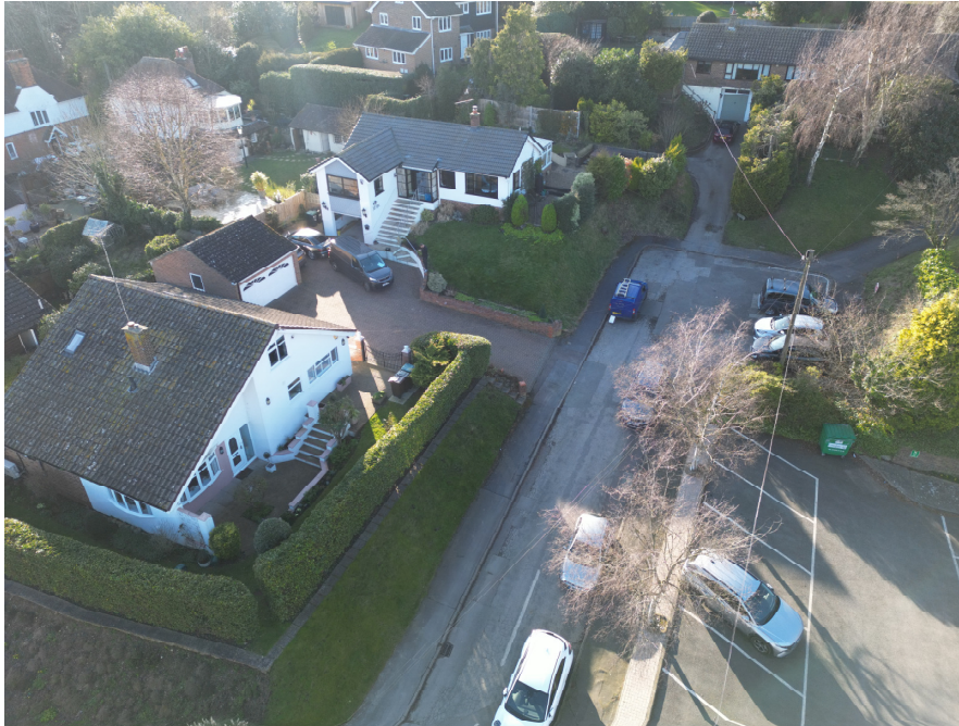
P00 – aerial view of site looking west
