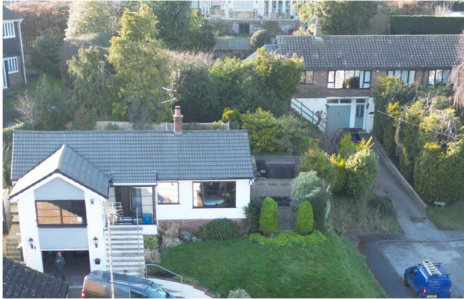
P007 – site context looking westerly
