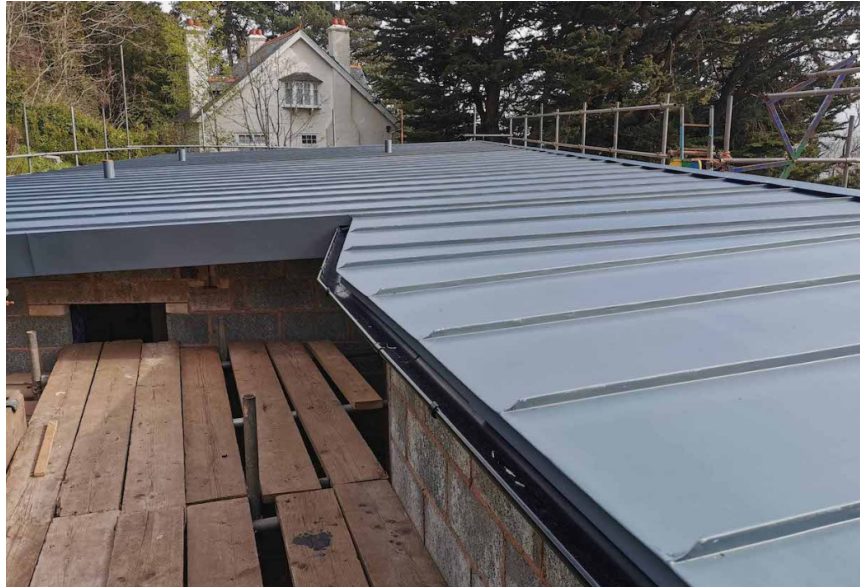
P003 – zinc standing seam roof
