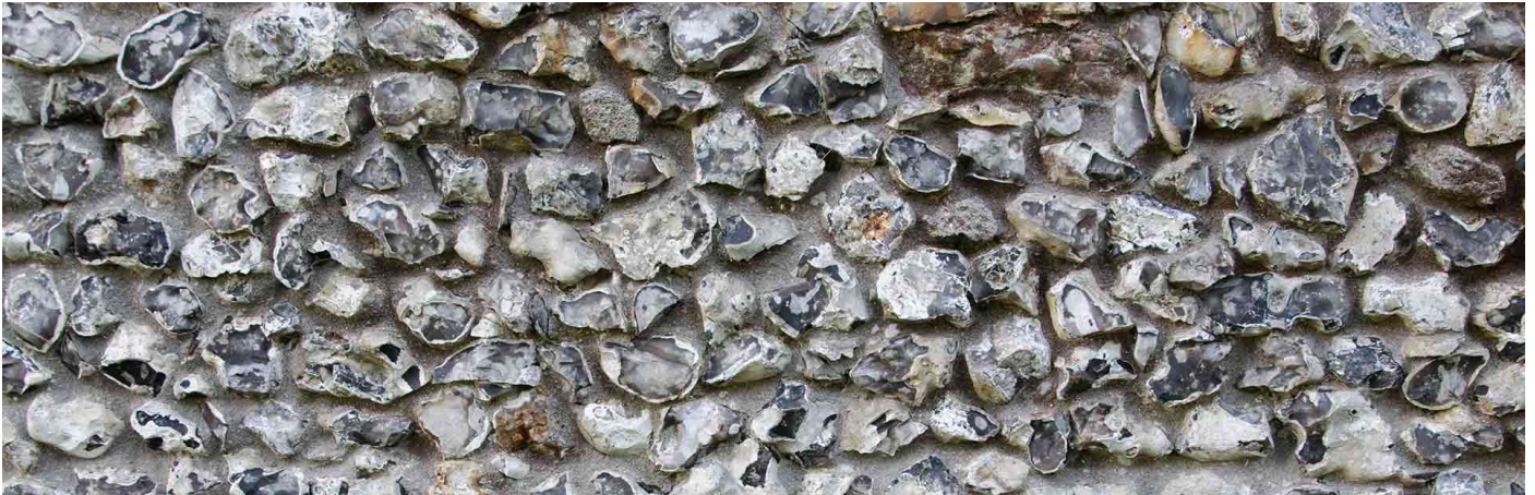
Flint stone walling to match the existing.
