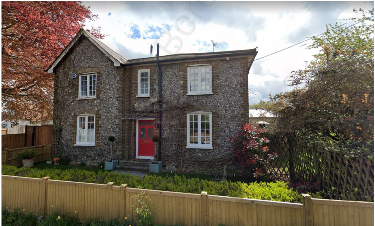
The Existing Dwelling - Seen from Main Street
