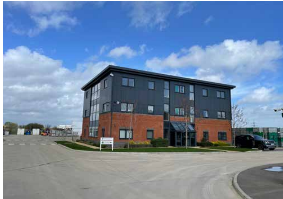
The existing O'Halloran & O'Brien office building has a brick base with cladding panels to the upper floors and pronounced overhanging eaves roof
