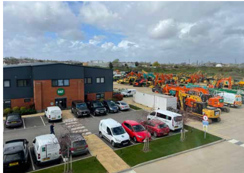
The existing B & T workshop and office building, with construction plant equipment in external storage areas behind. Westcourt Marshes are visible beyond the industrial park boundary.
