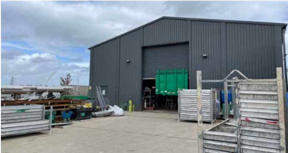
An additional storage building
