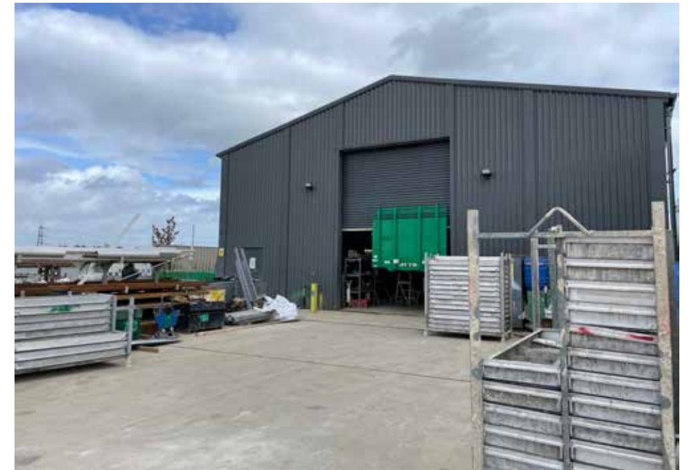
A storage facility in the North of the site provides protective cover to stored equipment.
