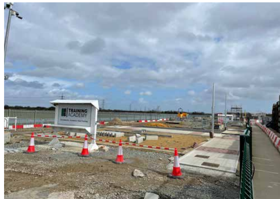
External areas of the Training Academy provide on-site experience which boost skills and employment opportunities. Westcourt Marshes are visible beyond the fence at the edge of the site.
