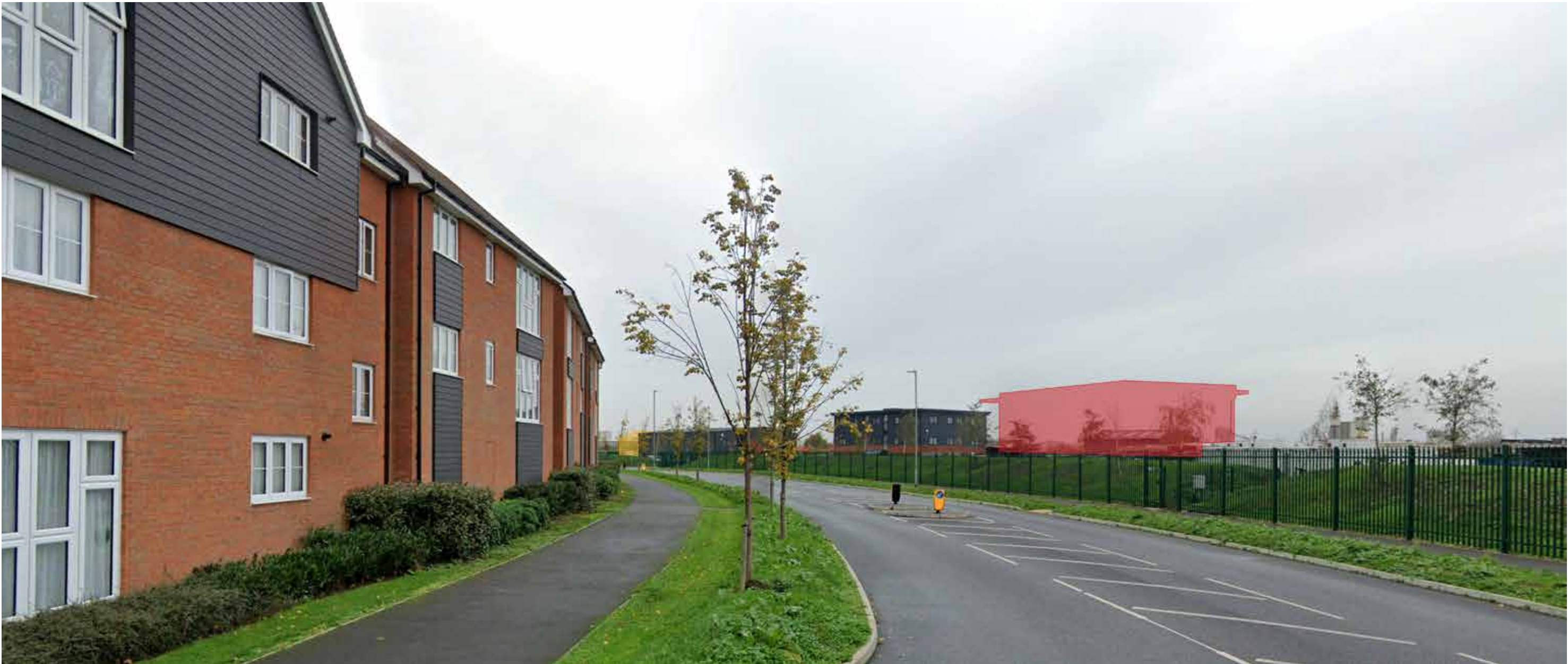
View 3: View from near the junction of Dalefield Way and Saltun Close looking North West.
