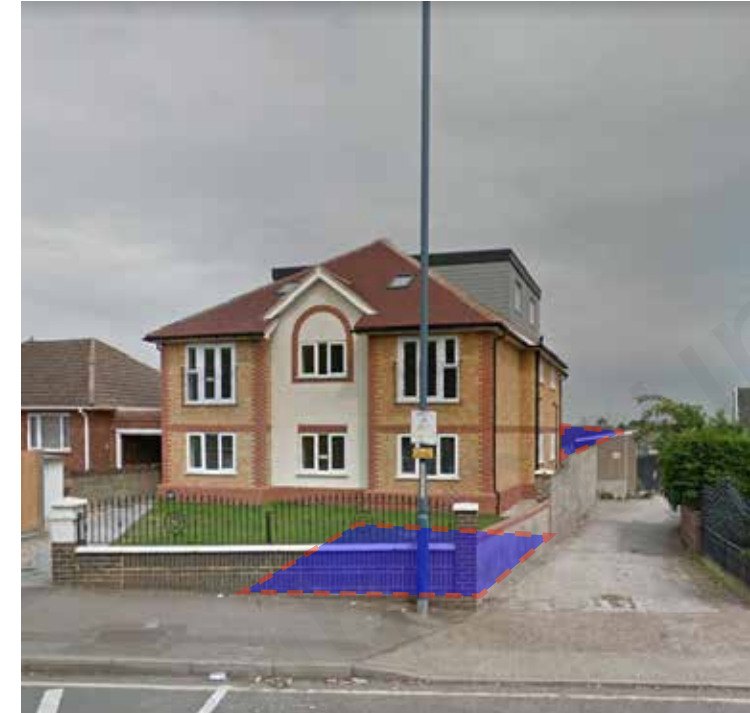
Photograph of 55 Rochester Road existing flats. Areas with proposed changes highlighted in blue.
