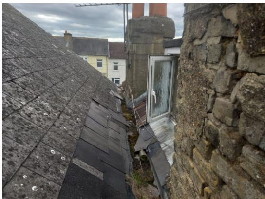
Photograph 03: Existing Roof to 57 Sun Lane
