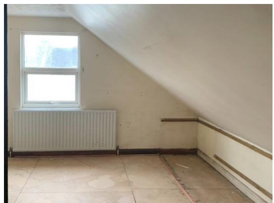
Photograph 04: Existing second floor rear bedroom
