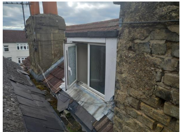
Photograph 02: Existing Dormer to 55 Sun Lane
