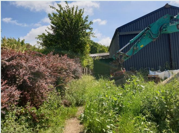
Overgrown area in south of site
