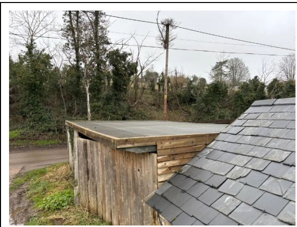
Photo 9: Building B2, timber building
