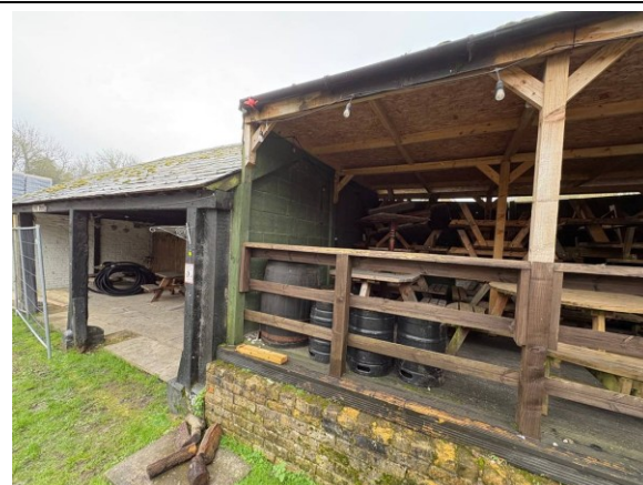
Photo 6: Building B1, open sided barns.
