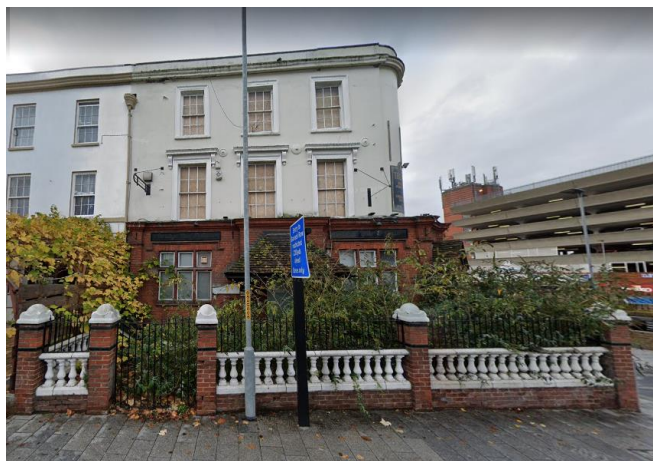
View from east on Stone Street
