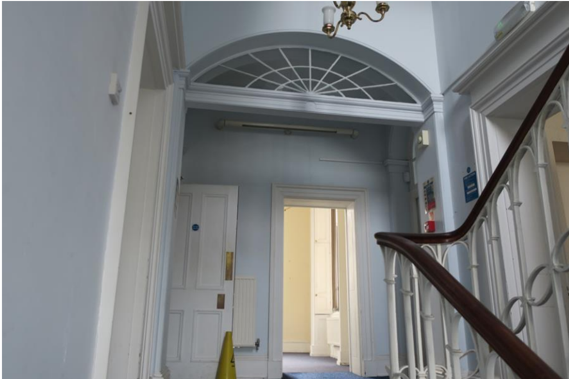
Fig 42 First floor landing on main staircase showing cast iron bannister and hardwood handrail, fanlight in archway to east-west corridor and doorcases into rooms off the staircase and landing, and beyond the arch to each side the modern firedoors in the inserted partitions.
