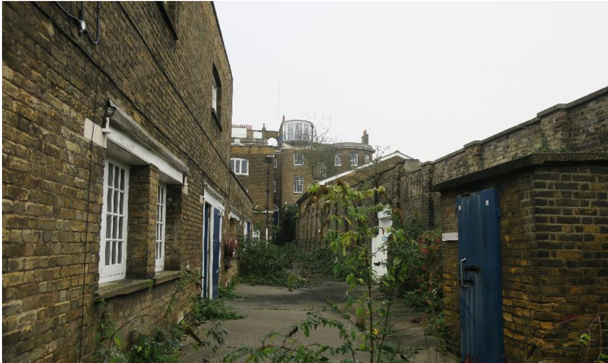
Fig 46 View up the passage of the other outbuildings
