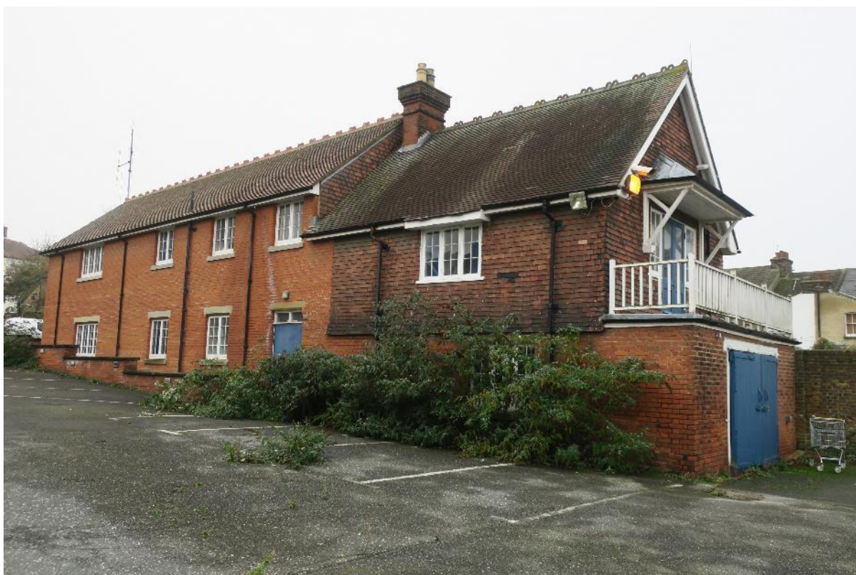
Fig 48 The former Coastguard station and later offices added to its south end, replacing an earlier small building.
