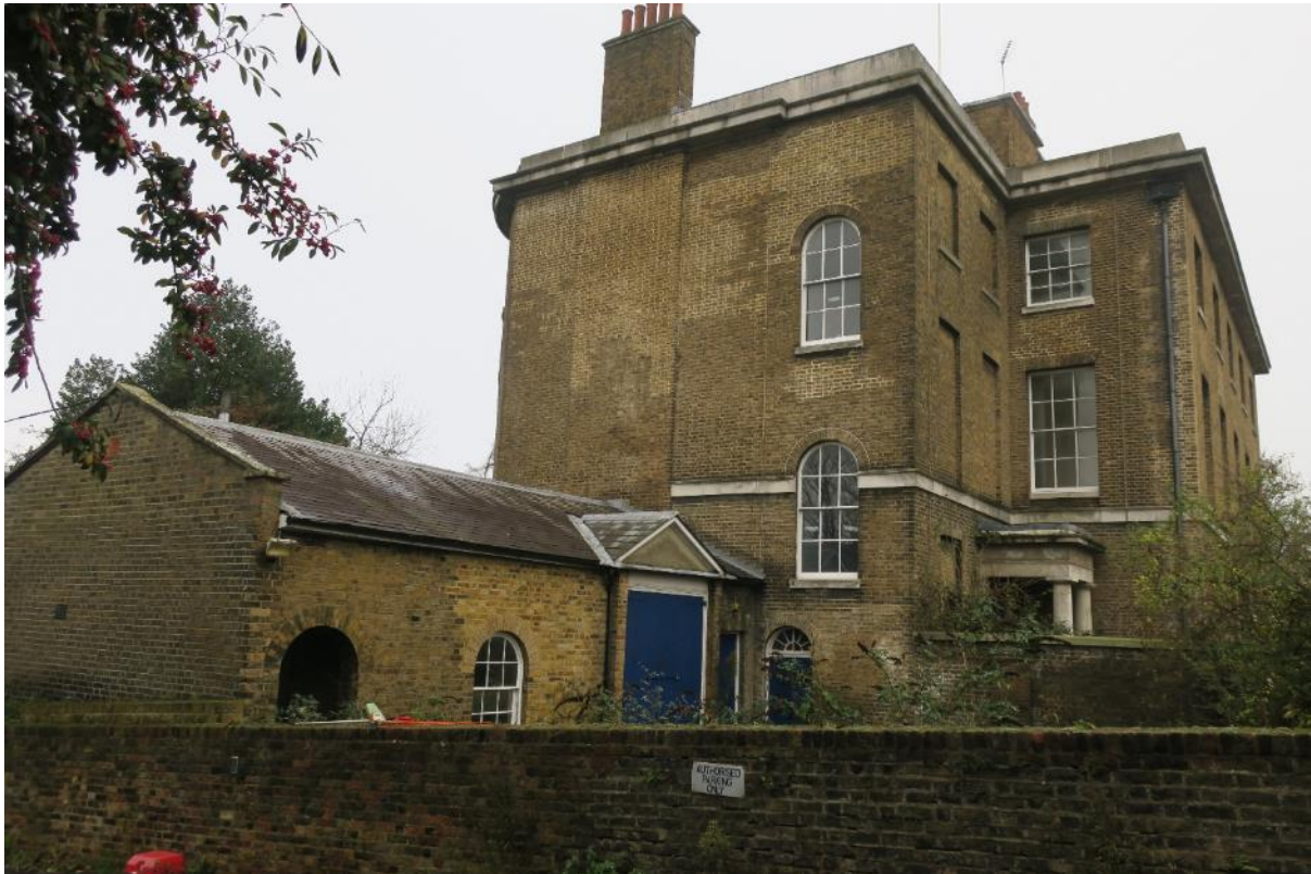
Fig 28 View from south west of main elevation of the Custom House, showing the coach house in the foreground with the areas of its front wall showing rebuilding
