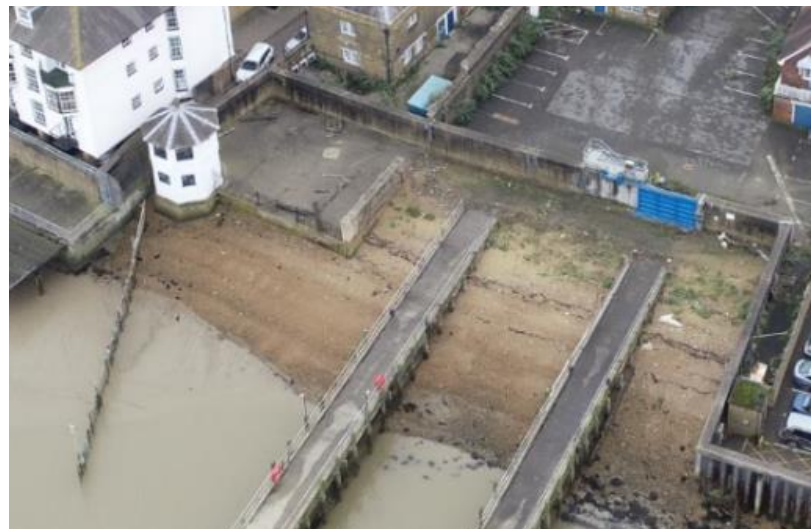
Photograph of Thames Riverside area, and flood defences.
