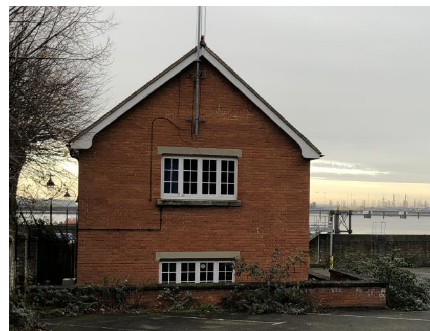
The rear Boathouse elevation.
