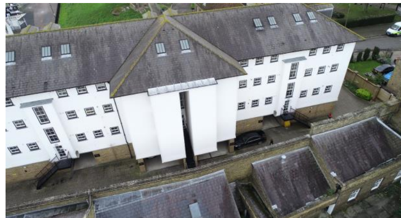
Photograph of Heritage Quay and Outbuildings
