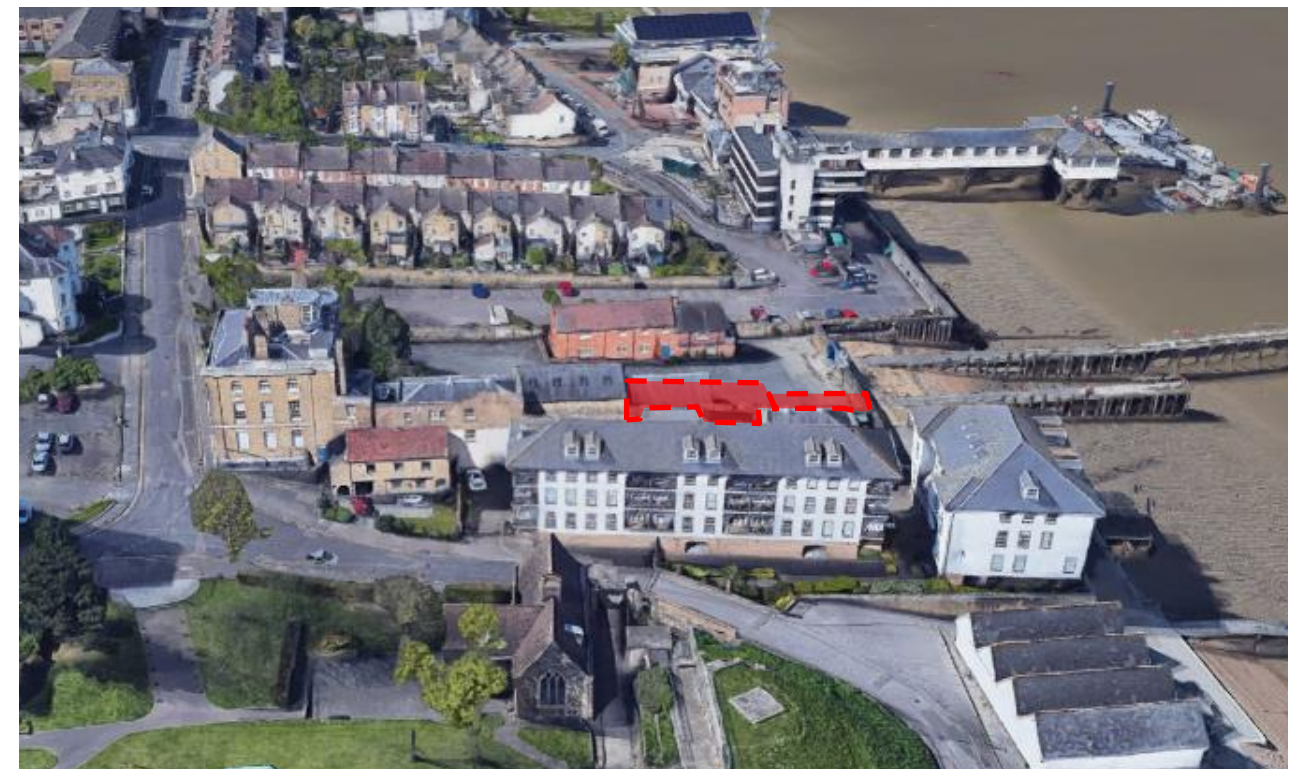
Current Photograph of site context with Royal Terrace Pier
