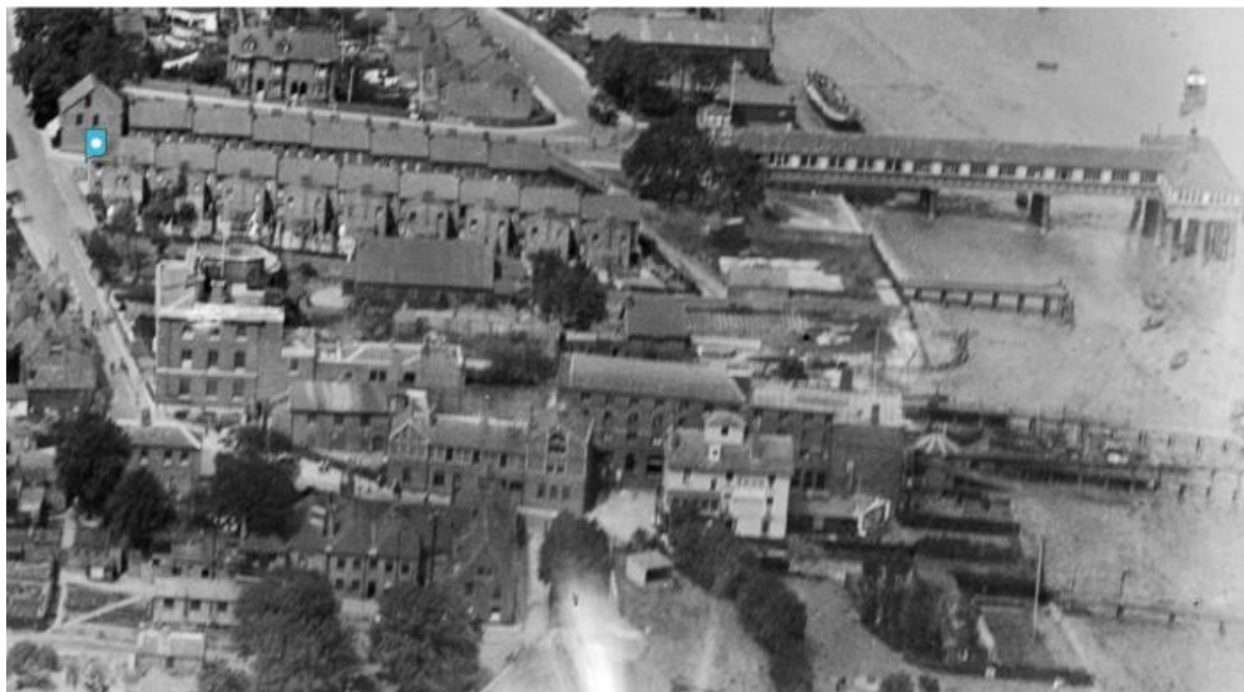
1920 Photograph of site context with Royal Terrace Pier
