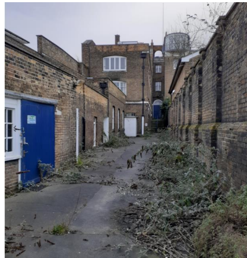
Photograph of historic access route, looking south.
