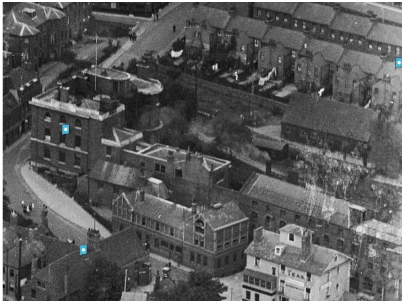
1920 Photograph of bonded warehouses along flank wall.
