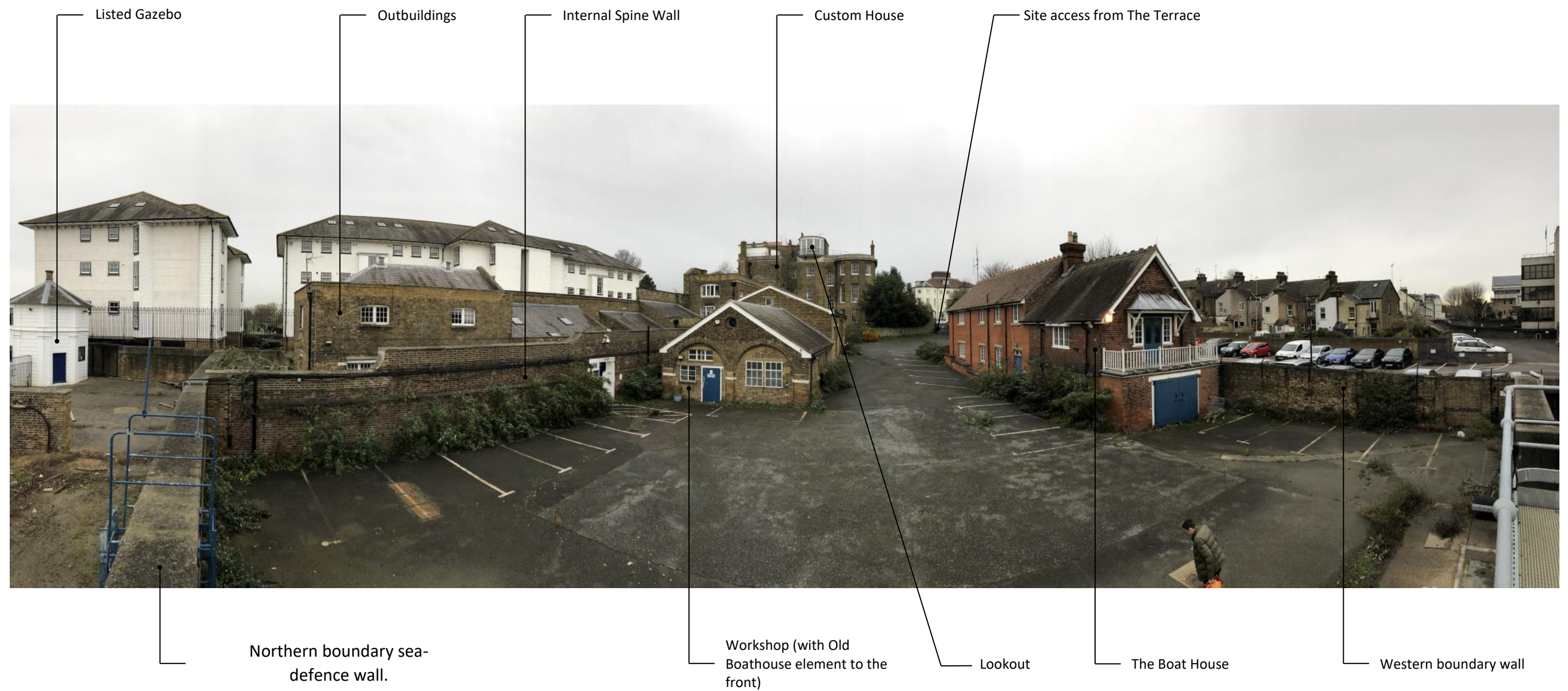
Panoramic view looking south from the sites northern boundary.
