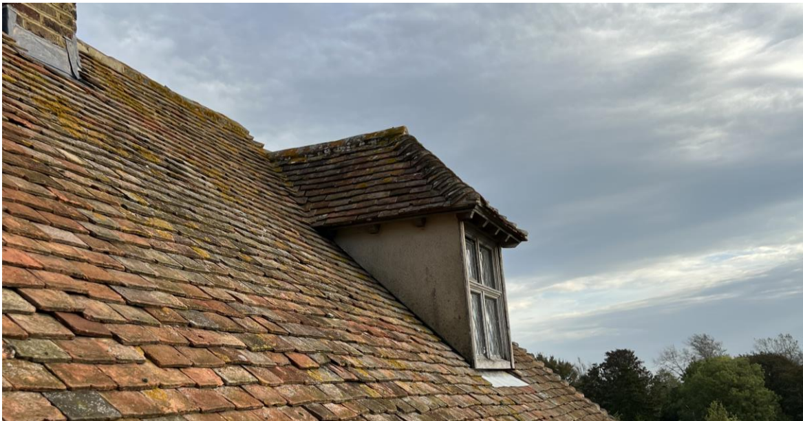
The above is a historic example of a rear dormer on a grade II* listed building near Deal, a former farmhouse set in a rural location. This example shows the hipped tiled roof with plaster dormer side-cheeks, this is a dormer for one of the attic rooms.
