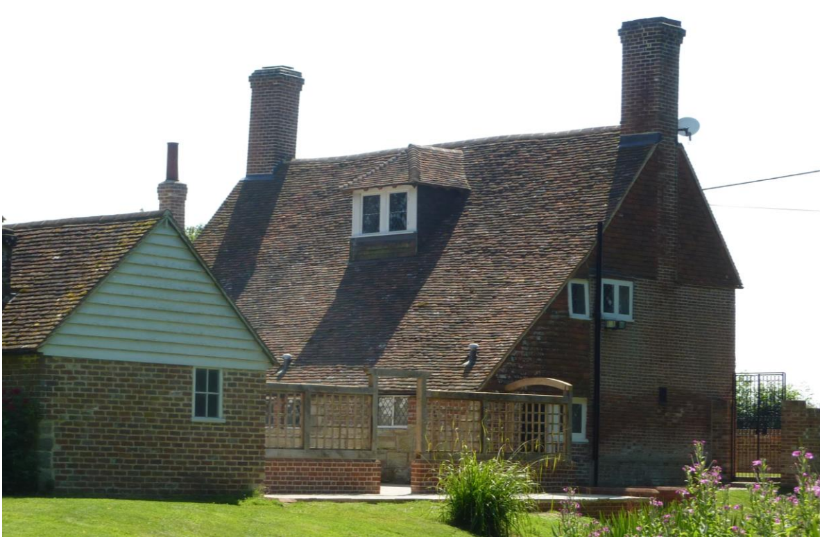
The above is a historic example of a rear access dormer on a grade II listed building, a former farmhouse set in a rural location. This example goes from eaves-beam and close to the ridge with an outshot below the dormer.
