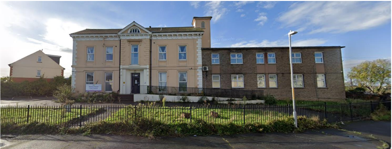
Figure 1: Existing street scene showing site frontage
