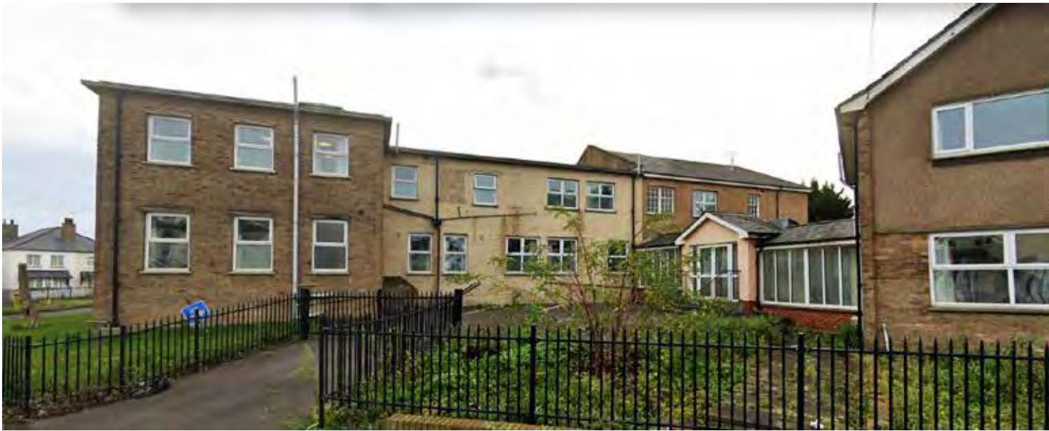
2 Side view of existing care home on site (secondary access)
