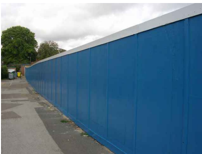
TREE PROTECTIVE Site hoarding
