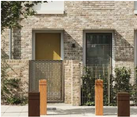
Brick wall with Metal Meshing Fencing
