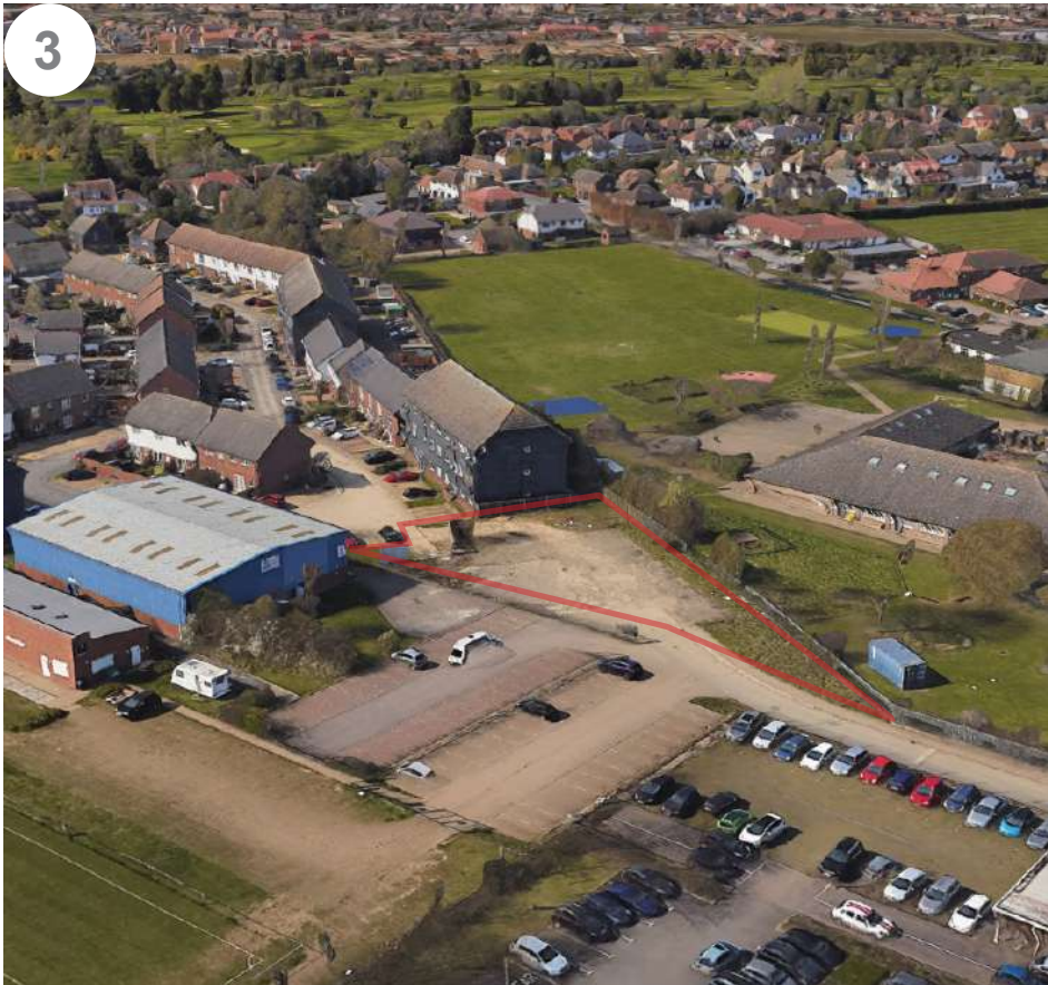
Aerial view looking north west
