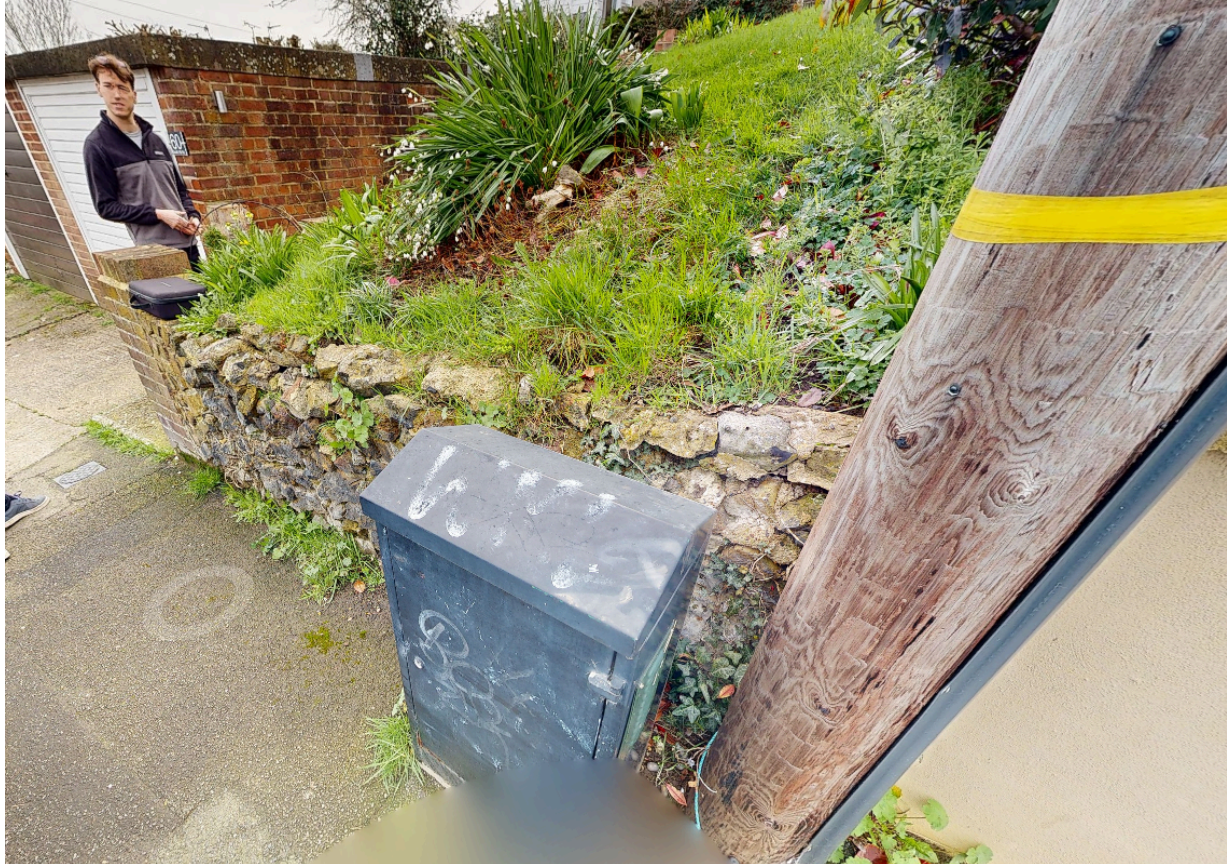
Image: Existing Burr Brick Wall which requires reconstruction screened by parked cars, feeder pillar and telegraph pole
