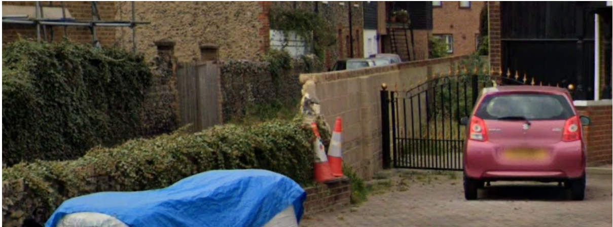
Figure 3: Street view image of the Site with particular focus on the as-built gate. (Source: Google Maps, April 2021)
