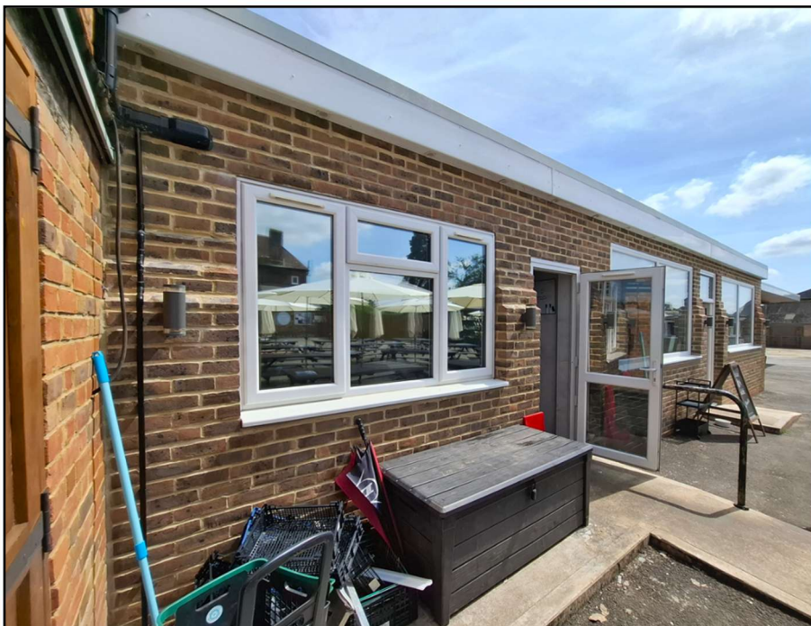
▪ BUILDING C: ELEVATION FACING THE INTERNAL COURTYARD.
