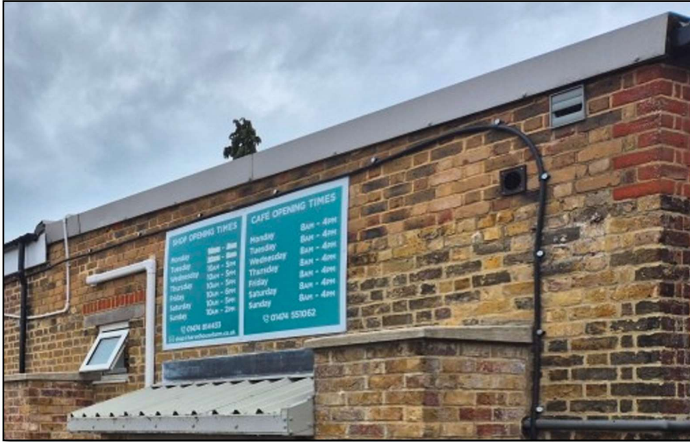
■ BUILDING B: NORTHEAST ELEVATION - EXISTING CONDITION
