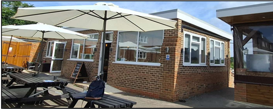
▪ BUILDING C: ELEVATION FACING THE INTERNAL COURTYARD.
