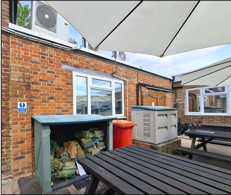
■ BUILDING B: ELEVATION FACING THE INTERNAL COURTYARD.
