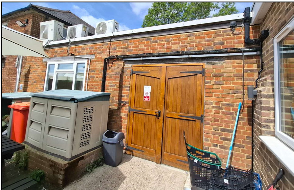
■ BUILDING B: ELEVATION FACING THE INTERNAL COURTYARD.
