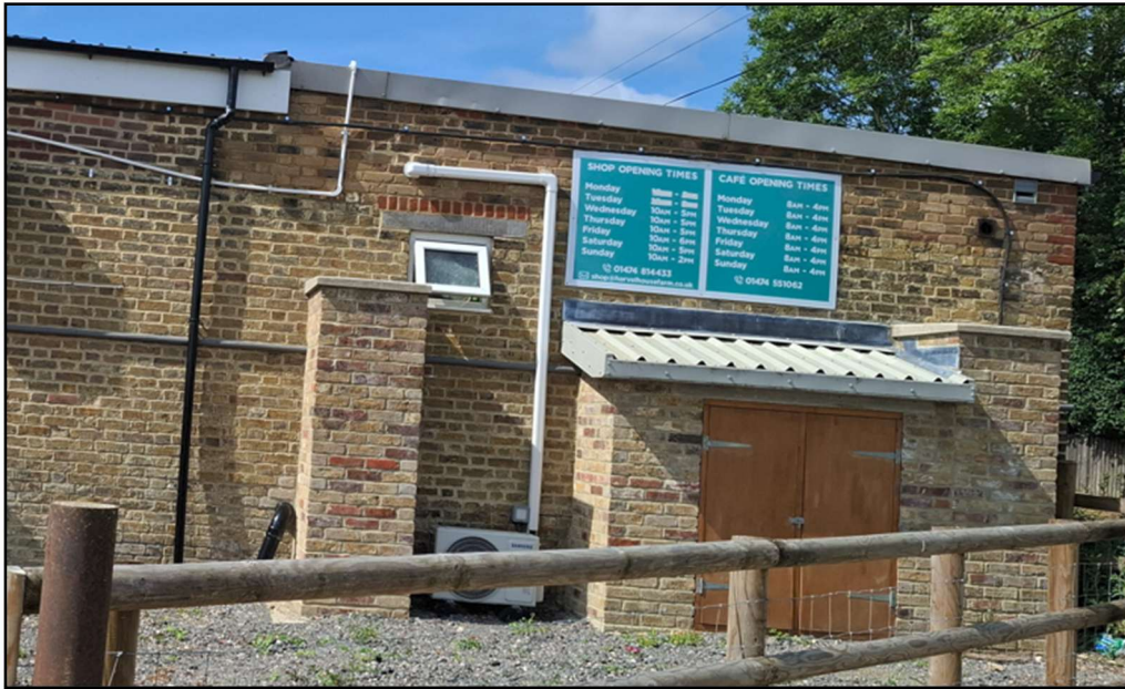
■ BUILDING B: NORTHEAST ELEVATION FACING THE CAR PARKING AREA- EXISTING CONDITION
