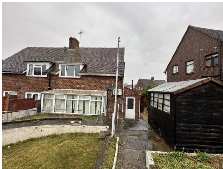
View of rear of the property
