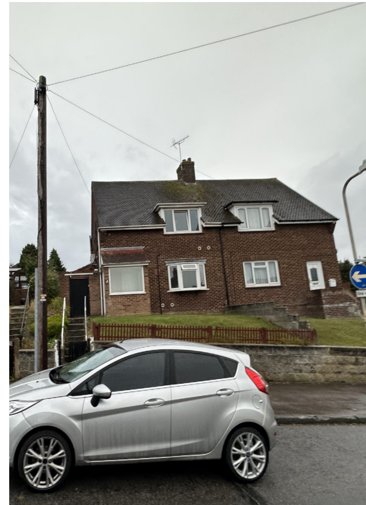
View of property from St George's Crescent
