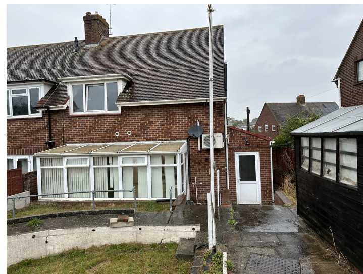
View of rear elevation
