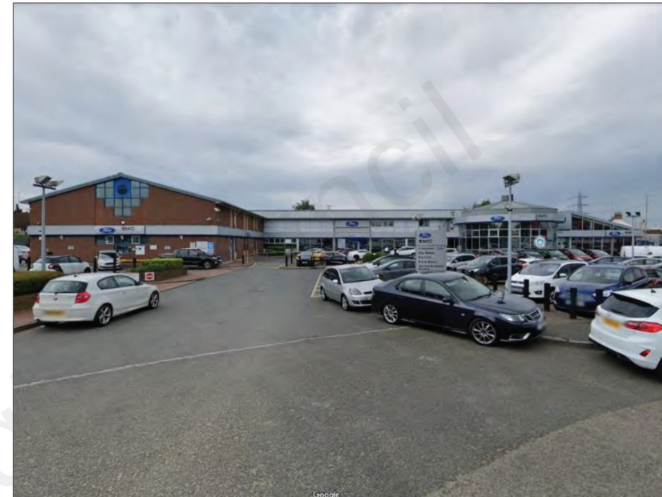
Plate 32) View of the SMC Ford Gravesend building located in the southern section of the Site, facing west
