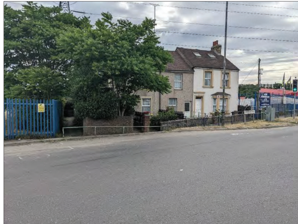
Plate 34) View of the three, 19th century terraced houses located on Lower Road, facing east
