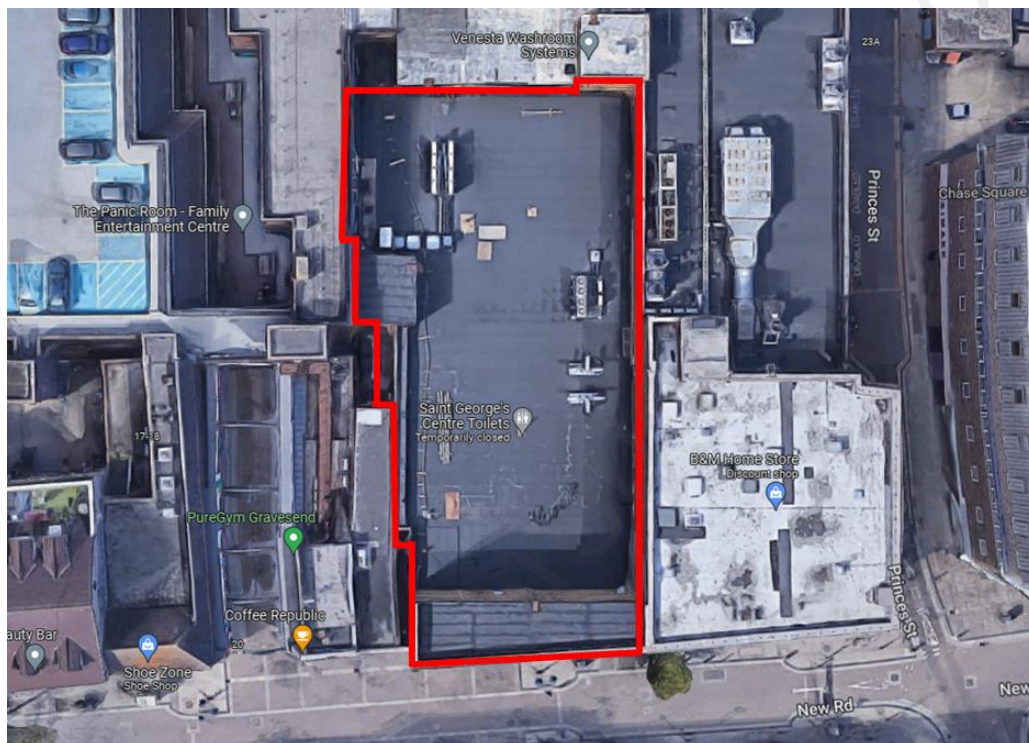
Figure 1 – Aerial view of application site (marked in red)
