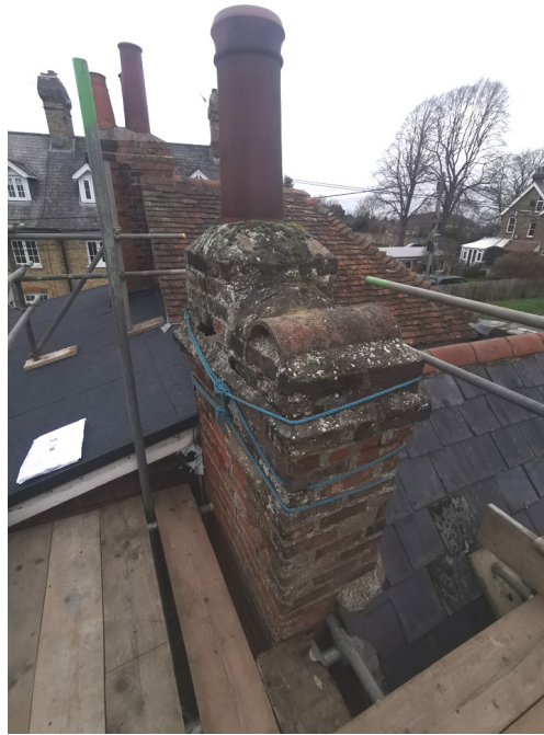
P008 – south west detail of chimney
