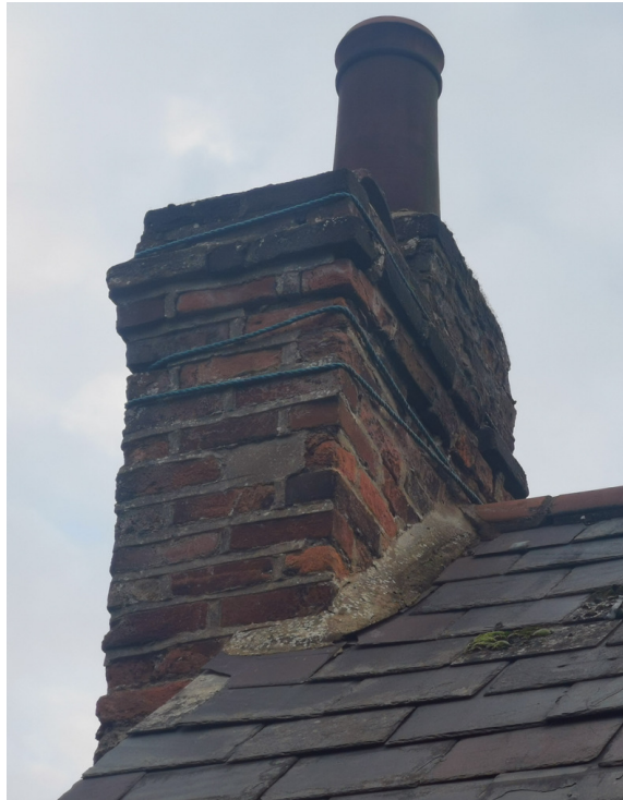
P003 – west face of chimney
