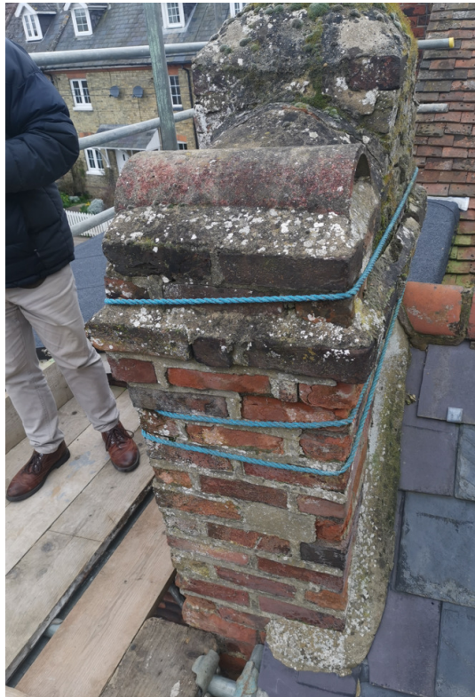
P005 – west face of chimney
