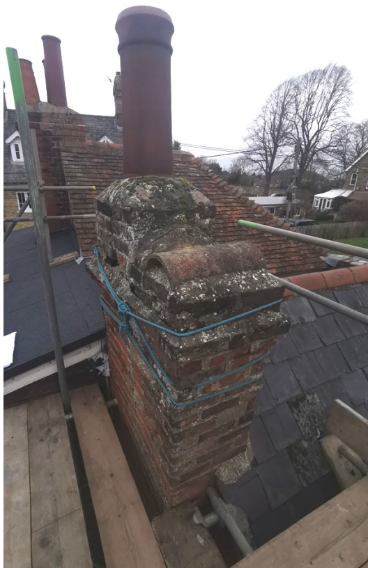
P006 – south face of chimney
