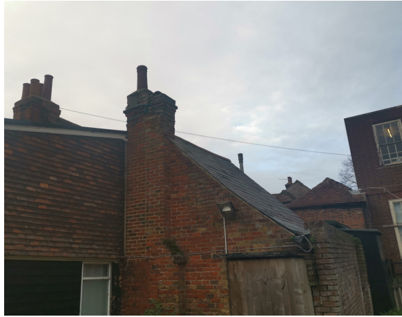
P002 – looking northerly from within school grounds
