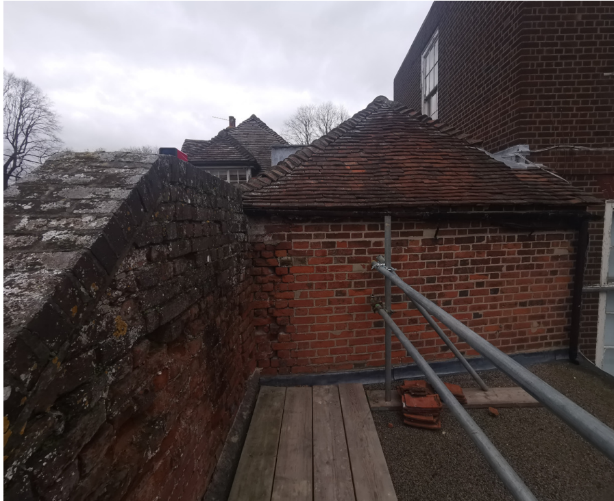
P004 – Internal side of parapet wall looking north
