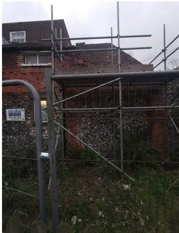
P003 – installed scaffolding
