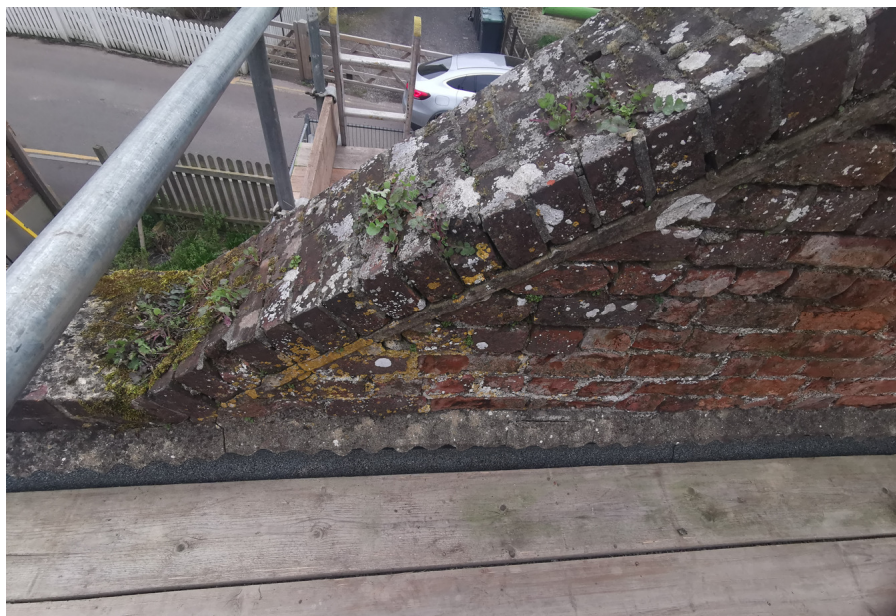
P005 – close up detail of internal side of parapet wall
