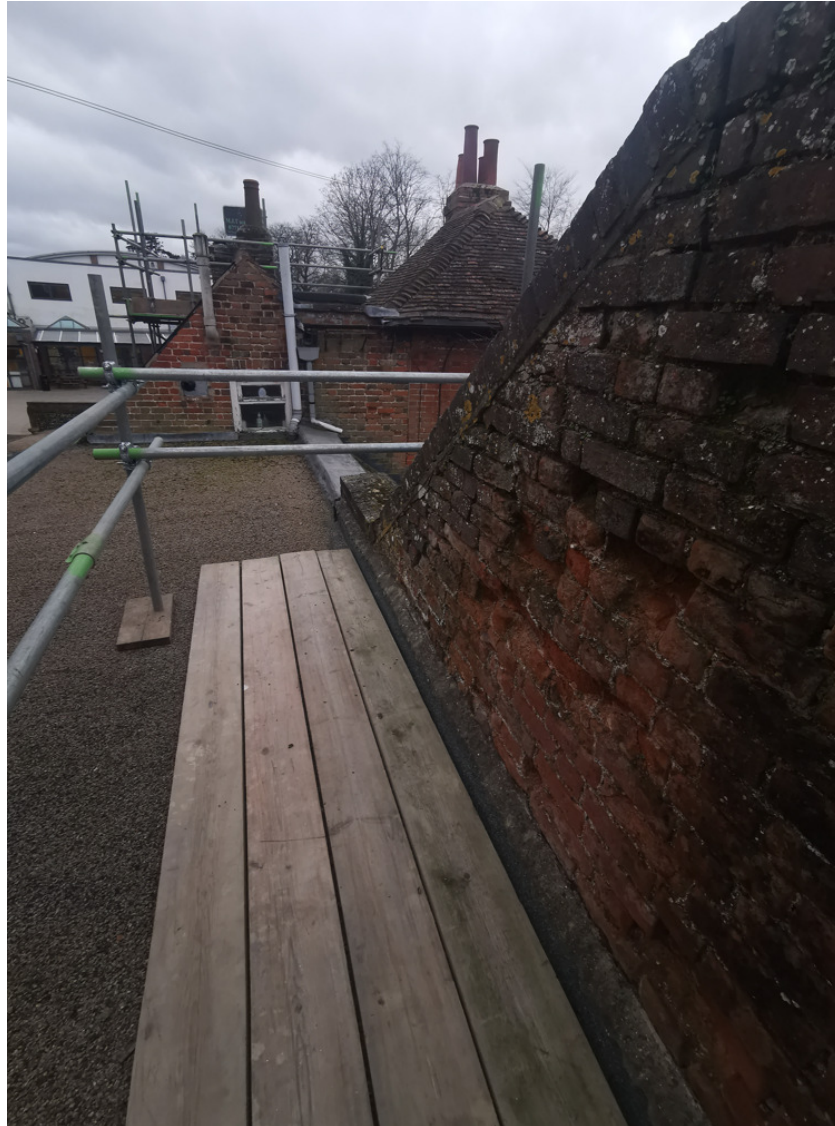
P006 – close up detail of internal side of parapet wall looking south
