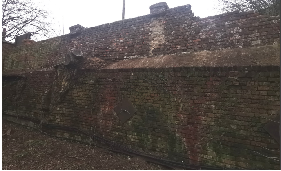
P001 – Internal side of existing fencing
