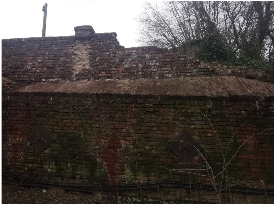
P001 – Internal side of existing fencing
