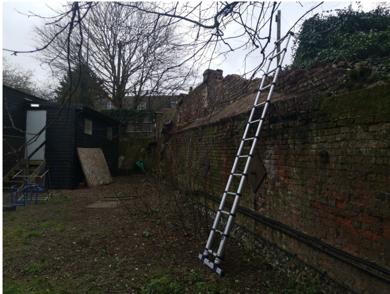
P001 – Internal side of existing fencing
