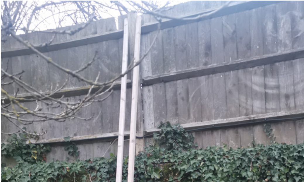
P001 – Internal side of existing fencing
