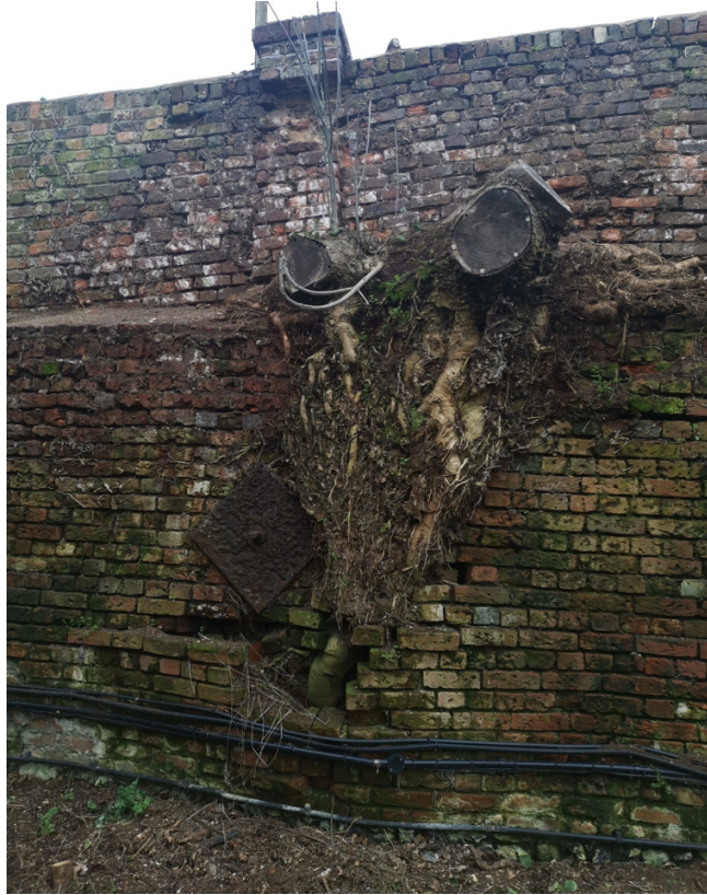
P001 – Internal side of existing fencing
