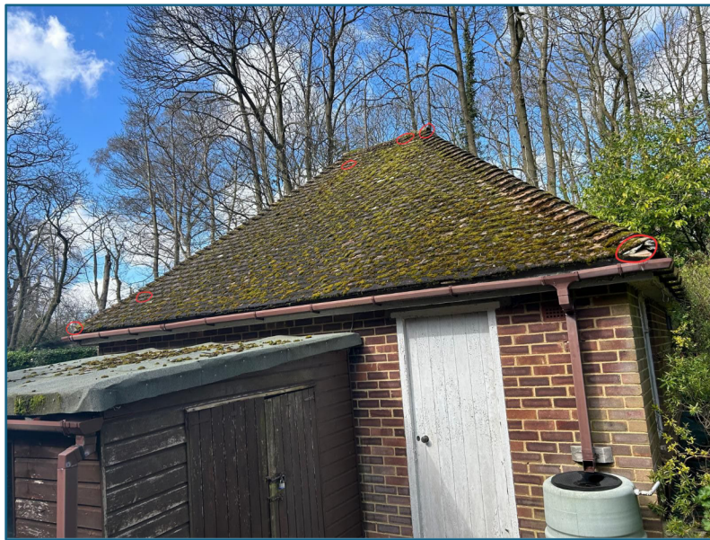
Figure 7: PRF visible on the south eastern facing elevation of the garage
