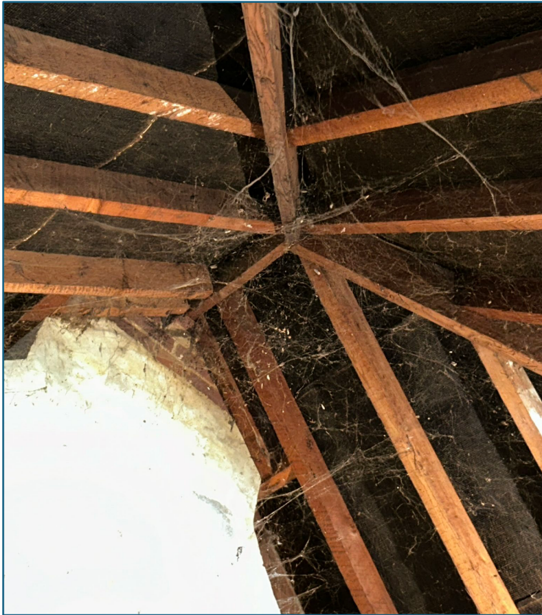
Figure 6: Internal loft area of the main house
