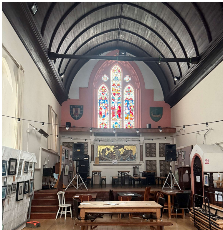
2025 Internal photograph of St Andrews' Arts Centre, depicting the vaulted, timber-lined, expressed-rib ceiling
