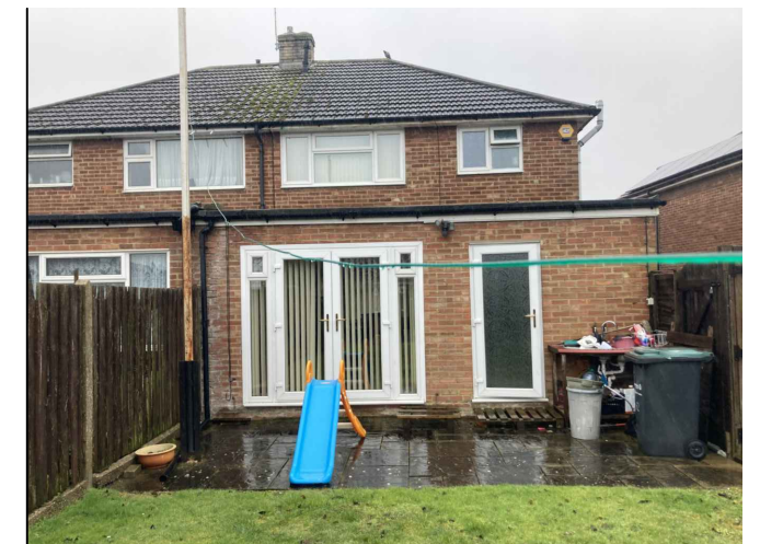
Photo 2: Existing rear elevation
