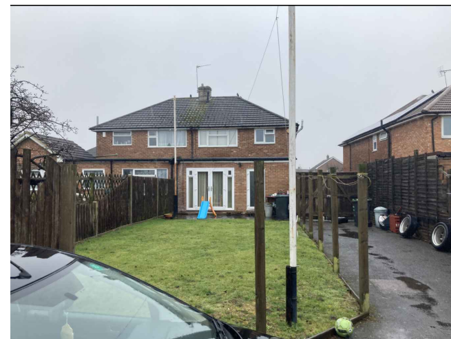
Photo 3: Existing rear elevation and neighbouring context
