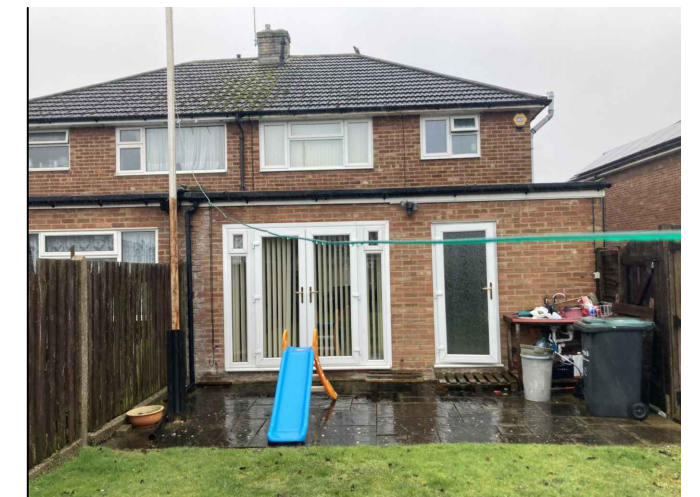
Photo 2: Existing rear elevation
