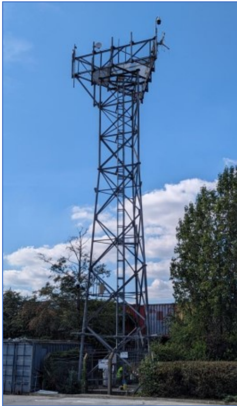
Figure 2: Existing tower at Denton Wharf
