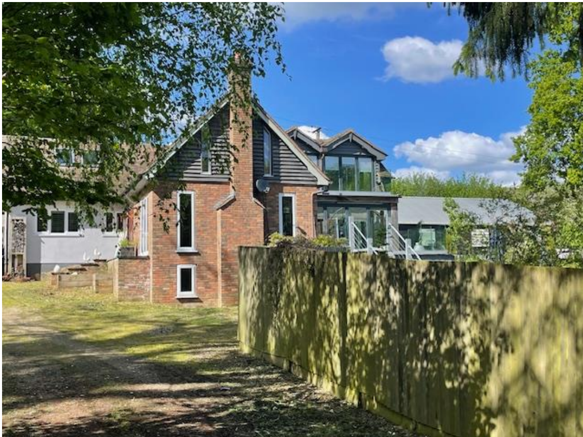
Primrose Cottage, Leywood Rd, Photo from Road, South Elevation, Now
