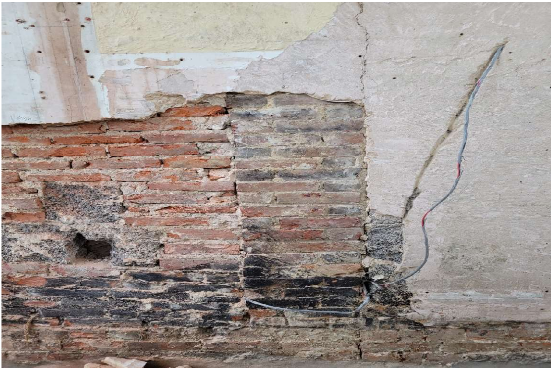
Rear Concrete Block Wall Ground floor
