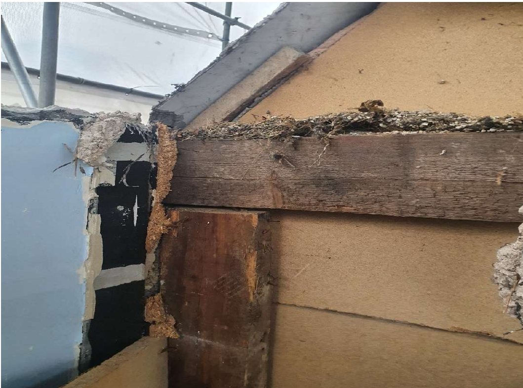
Internal Chipboard & Block Wall
