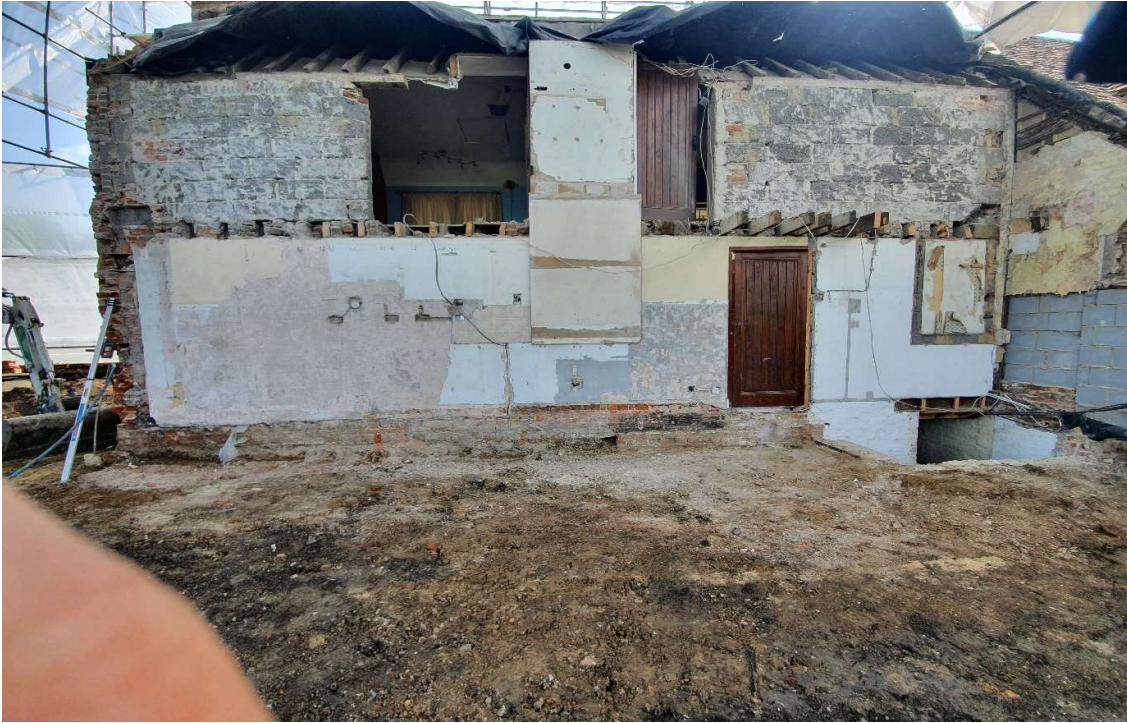
Rear Concrete Block Wall 1 st Flr
