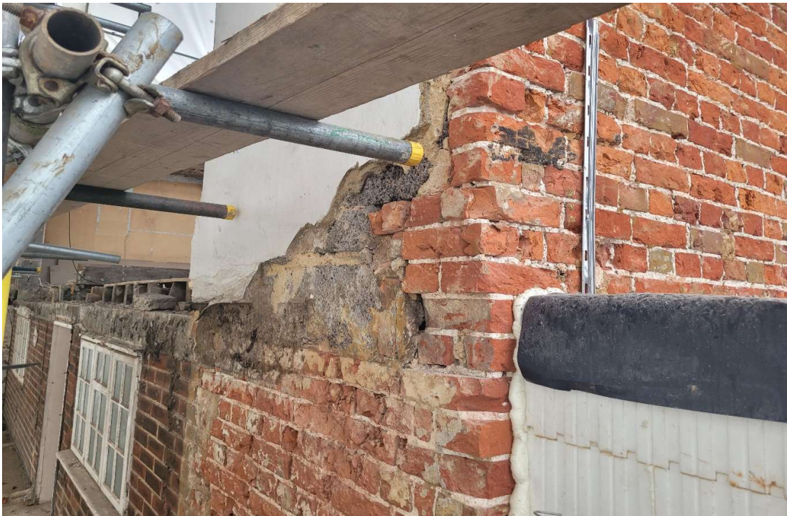
Front Concrete beam and 1 st Floor Concrete Block Wall
