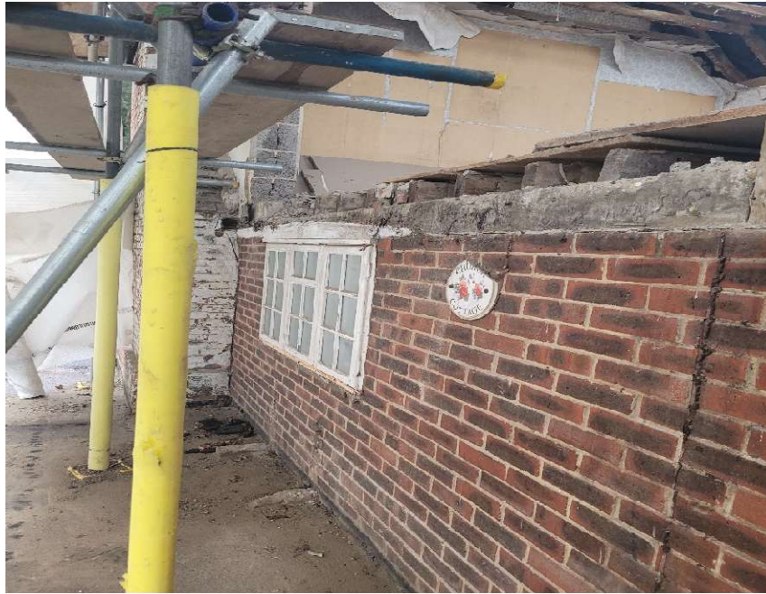
Front Concrete beam and 1 st Floor Concrete Block Wall
