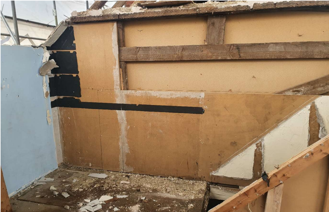
Internal Chipboard Wall
