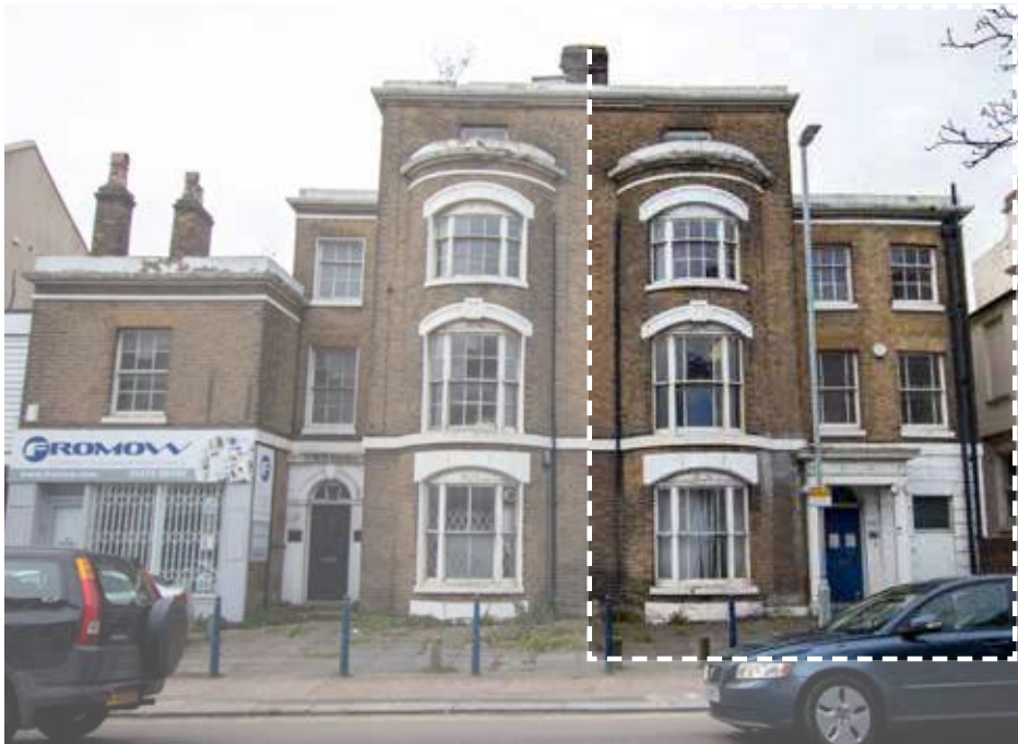
Left 197 Middle adjoining building 196 right 195 - application building
