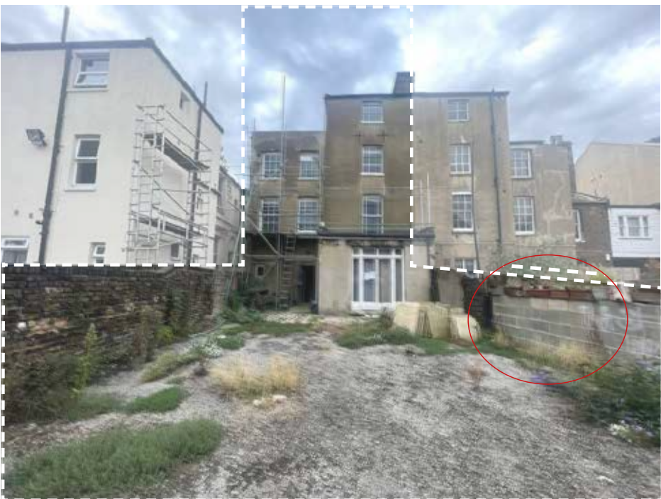
Left - 194 195 (centre) - application building Right no. 196 - adjoining building
