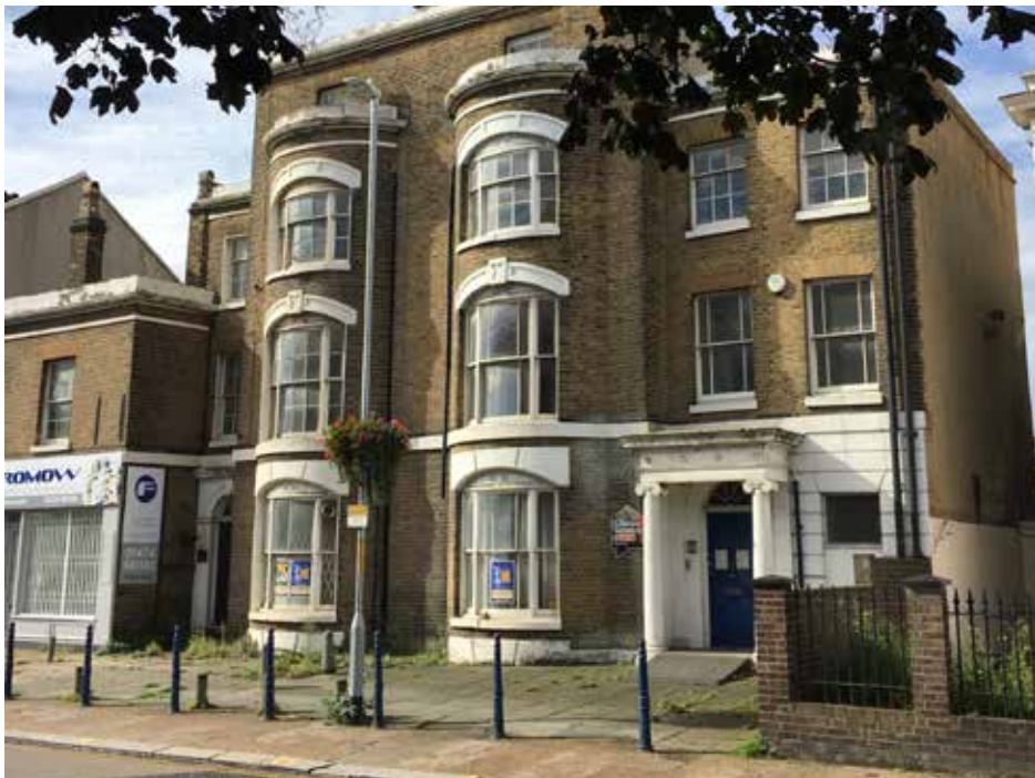
Left 197 Middle adjoining building 196 right 195 - application building
