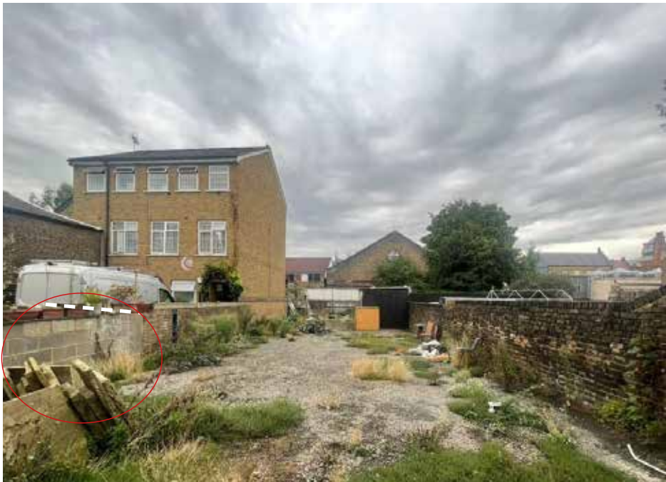
Fig 8: No. 195 - Rear view of garden and showing boundary wall block-work infill to no. 197, brick boundary wall to no. 194 and 3 storey, plus pitched roof neighbouring rear development flatted scheme no. 197A - image from Allsop Estate Agents A virtual tour of the property in its purchased form may be viewed here: https://drive.google.com/file/d/1VWYaaAt9YViaYi-4W_9rNcBWT0xyjIK/view
