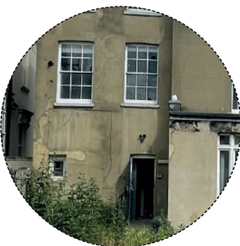
Rear Elevation North Wing Stucco
