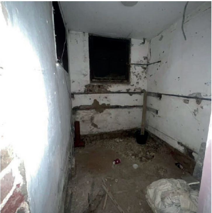
Fig. 42 Site photo: Existing environment (proposed bathroom LW03)
