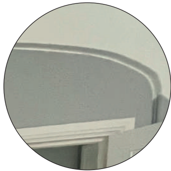
Evidence of arch left in situ infill partition to first floor
