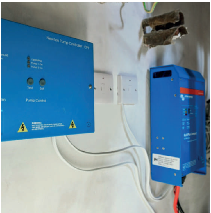
Fig. 44 Proposed inverter and pump controller
