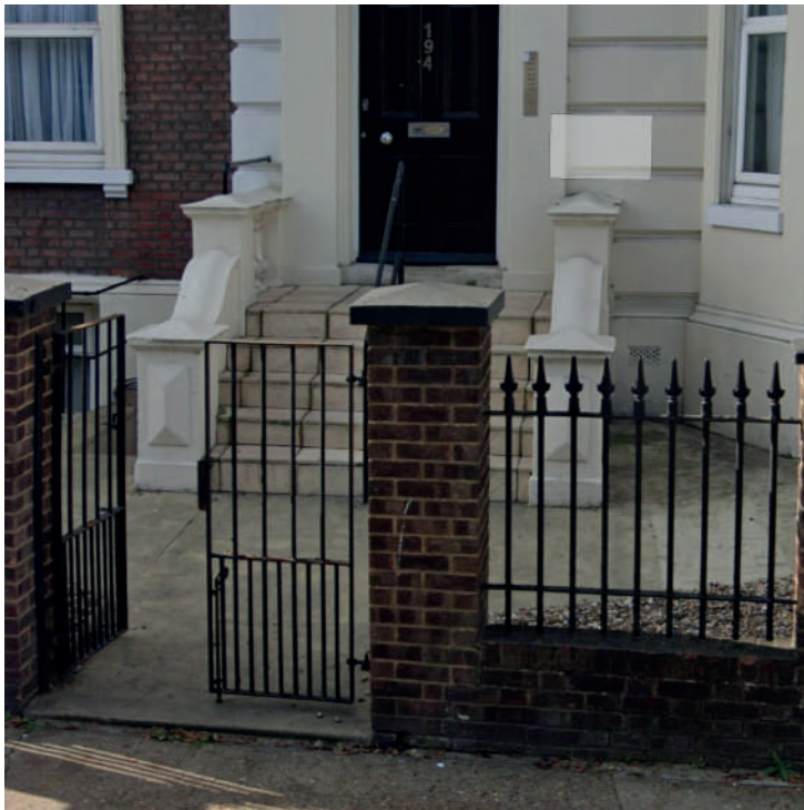
Fig. 47 Site photo: Neighbouring building 194 boundary treatment
