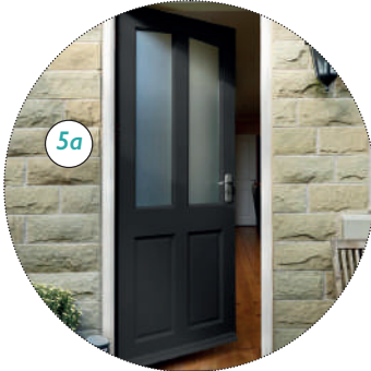
Central 1/2 glazed shaker door, sash tilt and turn white painted timber windows either side.
