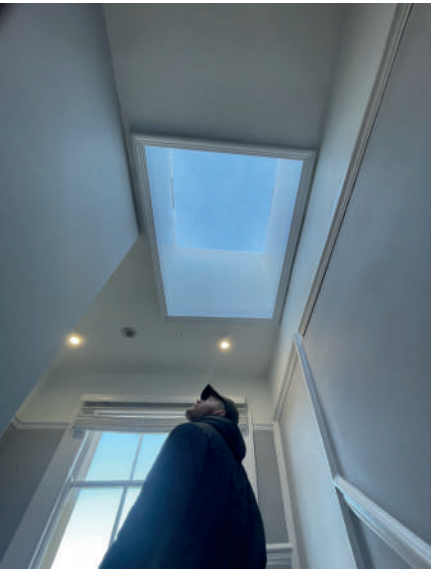
AOV formed over 2nd floor stairwell Fire Doors & Partitions
