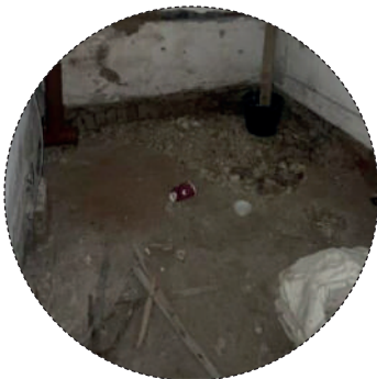
Stone flooring remains in situ
