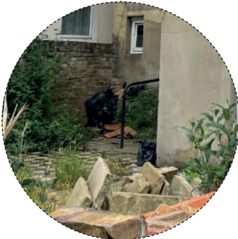
Stone slabs lifted, retained on site.
