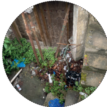
Previously in-filled light-well Opened up & revealed
