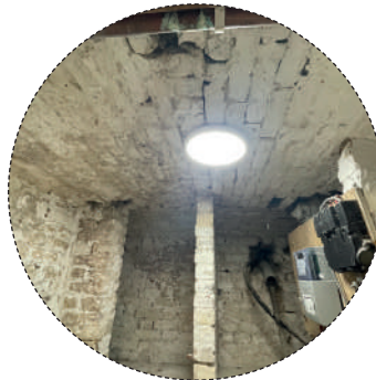
Original brick vaulted ceiling remains in situ.
