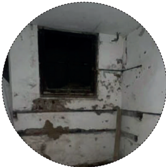
Light-well window remains in situ
