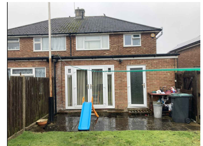
Photo 2: Existing rear elevation
