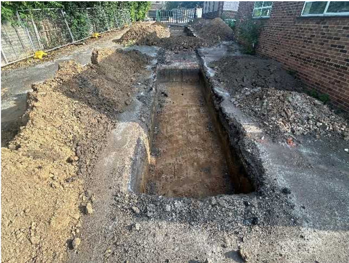
Photo 4. The Trench 1 from the south looking north
