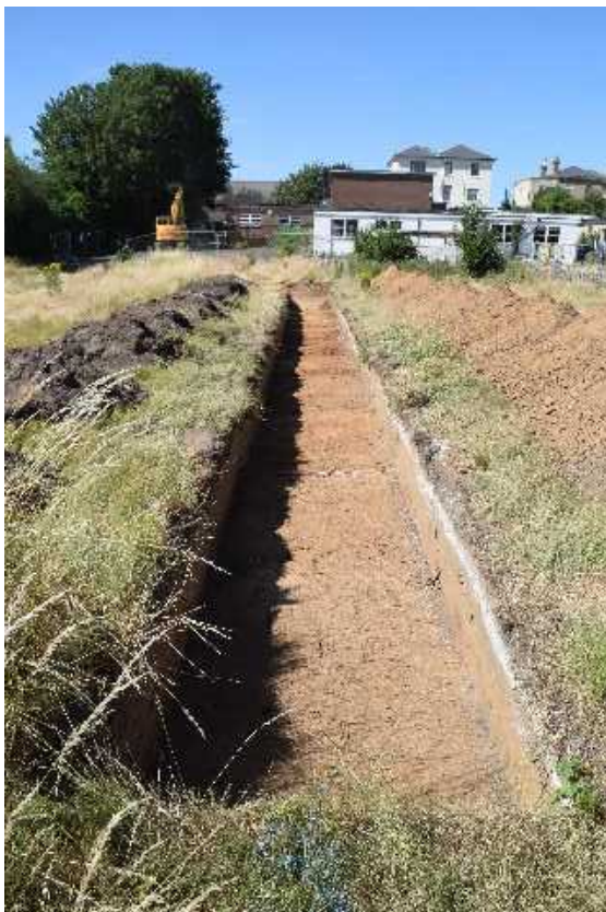
Photo 8. View of excavated Trench 3, looking north. Scale 1.0m
