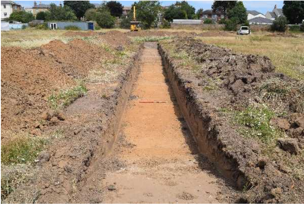
Photo 31. View of excavated Trench 11, looking south. Scale 1.0m
