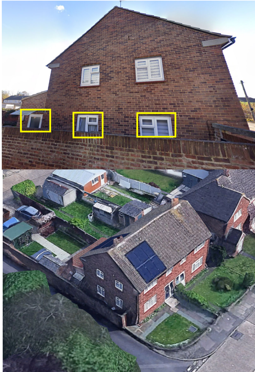
Figure 13. Google Earth images of 1 Everest Close (windows 156, 157 and 158 highlighted in yellow)
