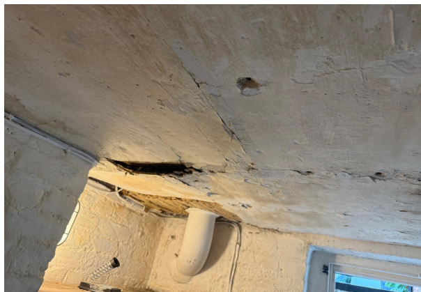
Photograph 4: Existing water-damaged lath and plaster ceiling.
