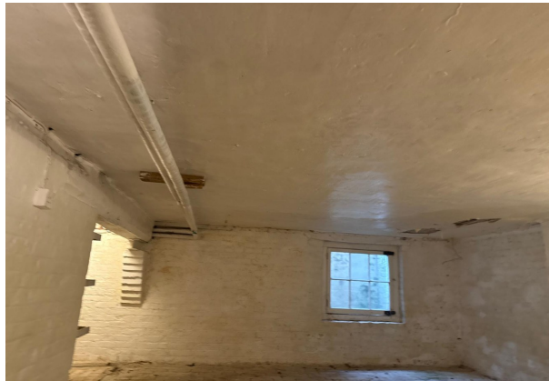
Photograph 4: Existing water-damaged lath and plaster ceiling.
