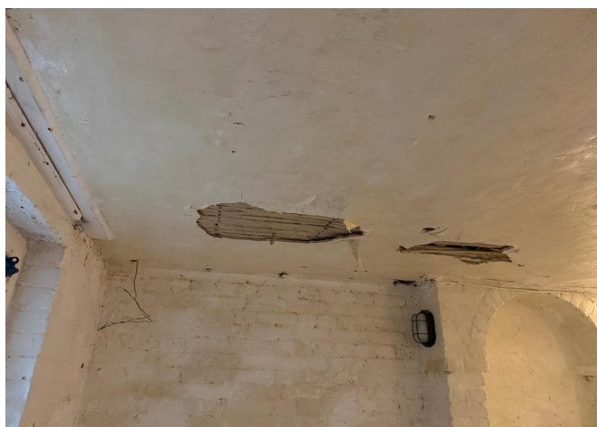
Photograph 2: Existing condition of the water-damaged lath and plaster ceiling at Jeskyns Court. Photographs show areas of cracking, plaster loss and exposed laths.
