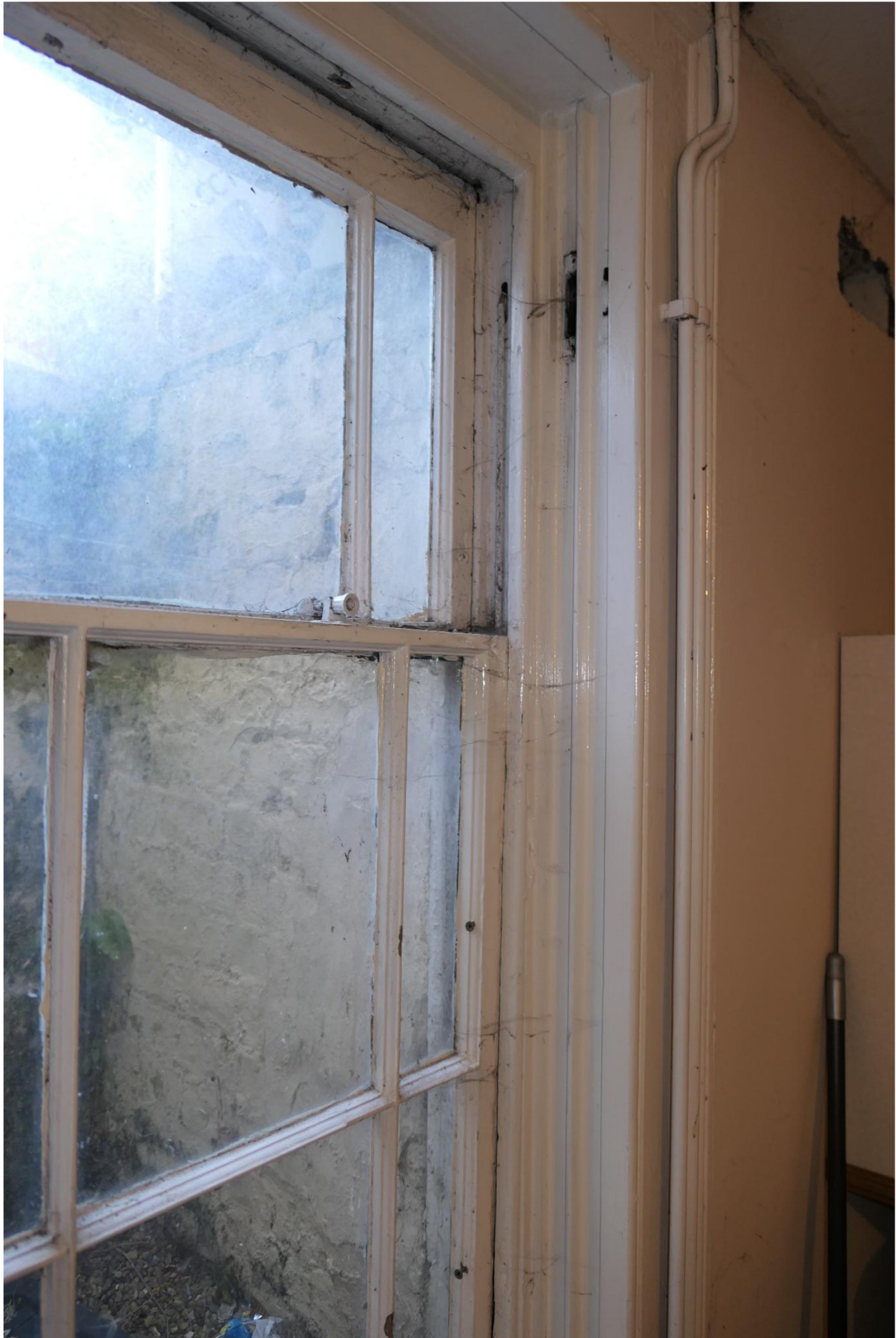
Photo 8: A detail of the window reveal at the rear basement room.
