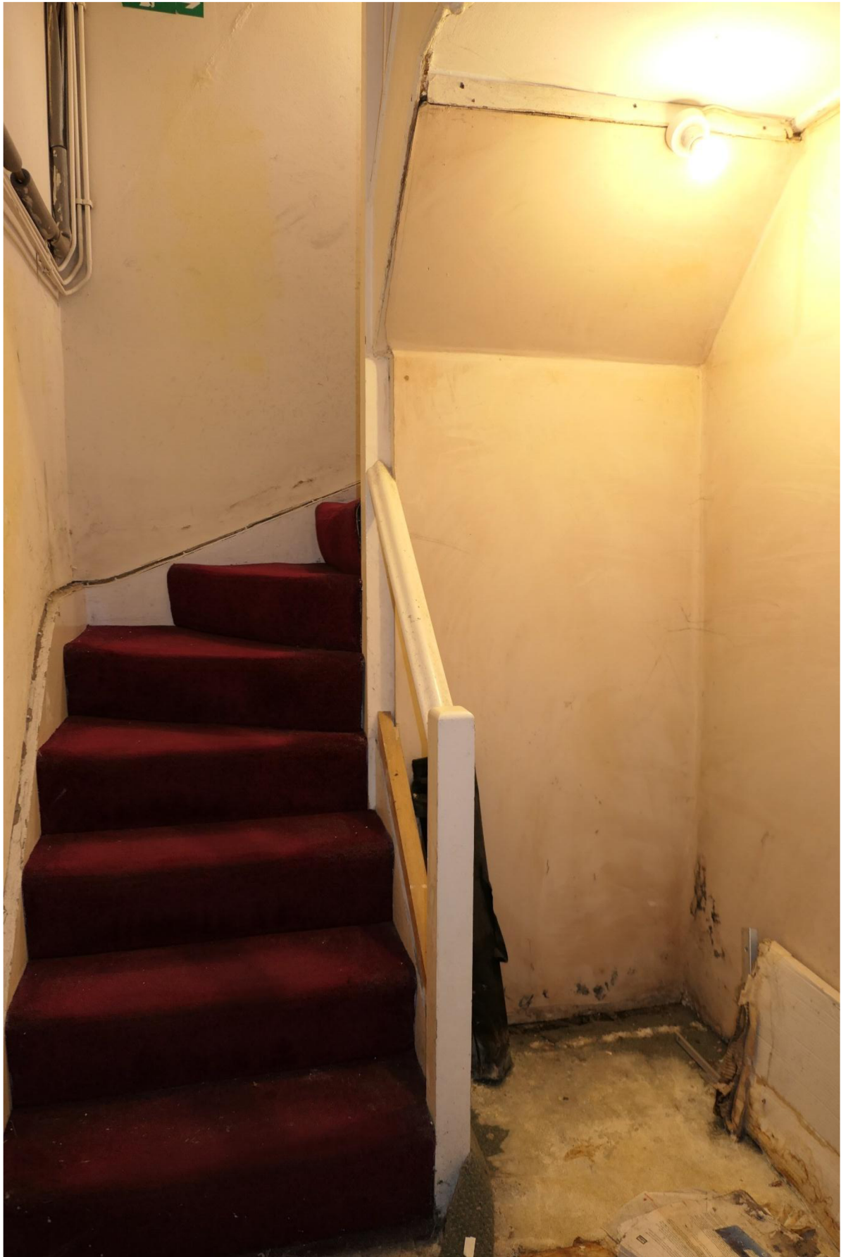
Photo 9: The basement stairs has been replaced.
