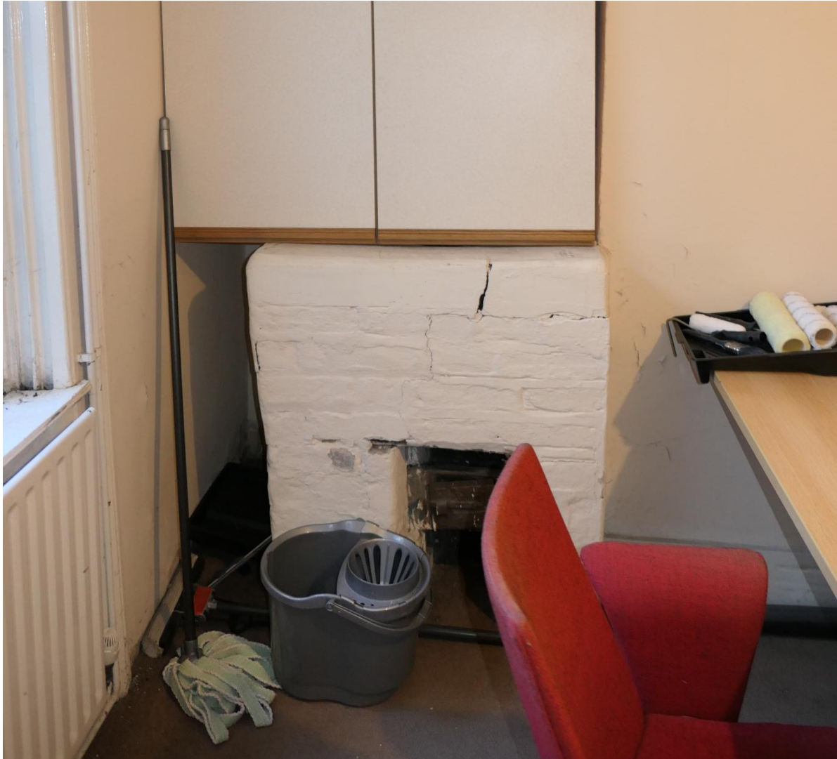
Photo 7: The little brick oven or stove-like structure adjacent to the chimneybreast in the rear basement room.
