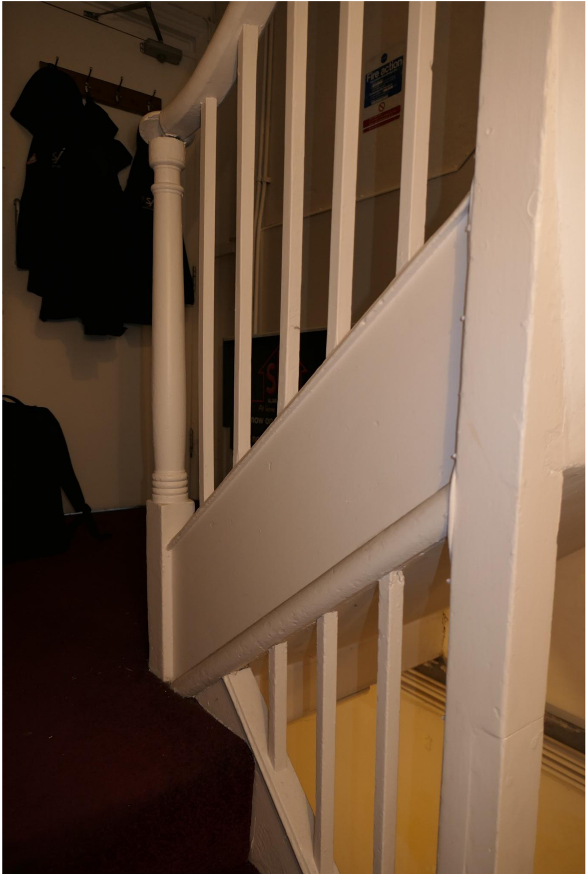
Photo 12: The staircase at the ground floor.
