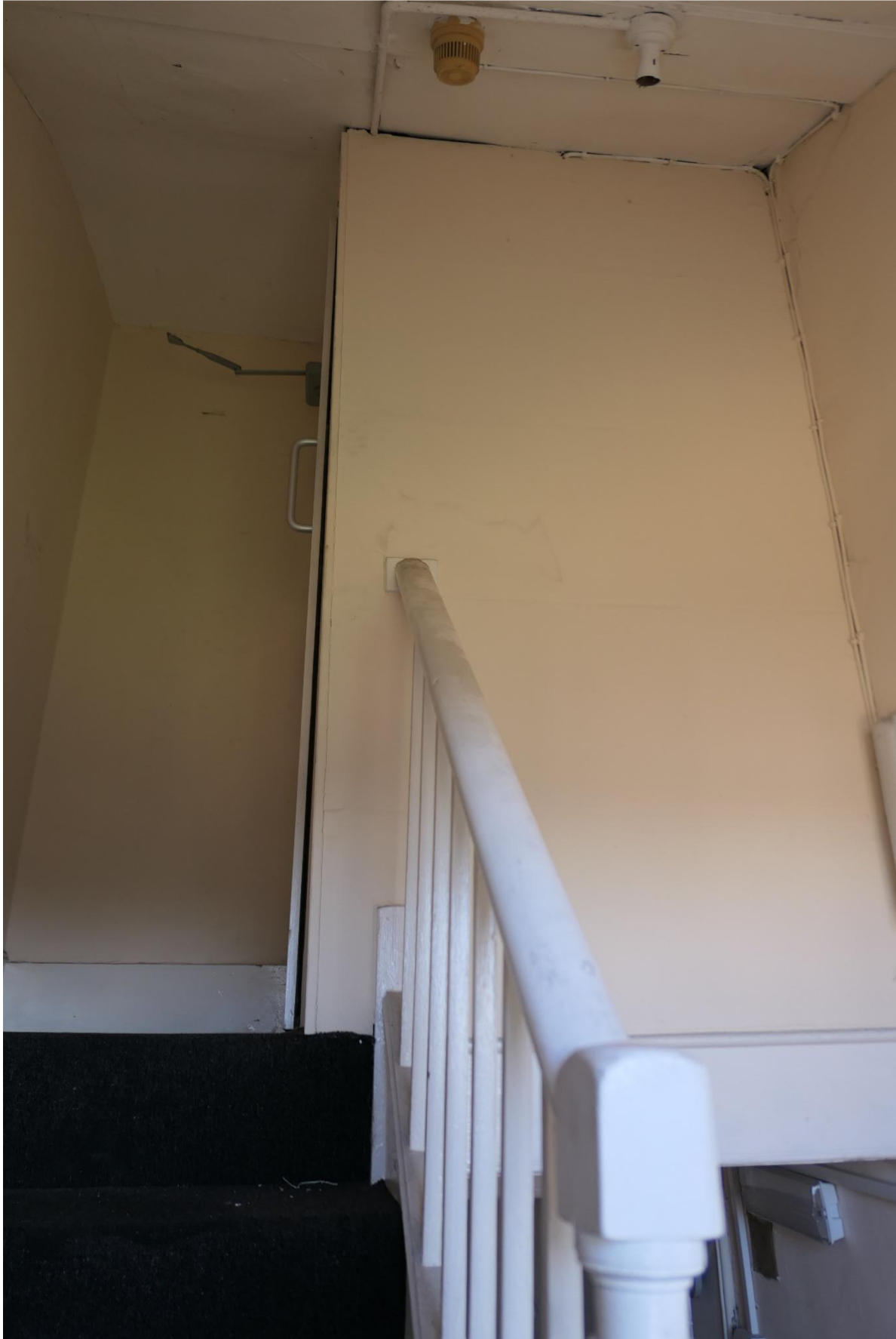
Photo 16: The staircase at the second floor has been truncated by a boxed lobby.
