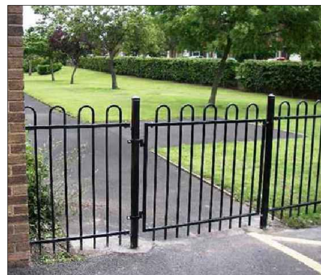
Proposed image of 1.2m high galv. and powder coated mild steel bowtop fencing and gate.
