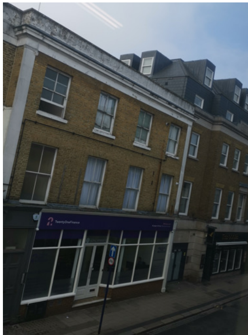
Fig 10 – adjacent building fenestration and detailing
