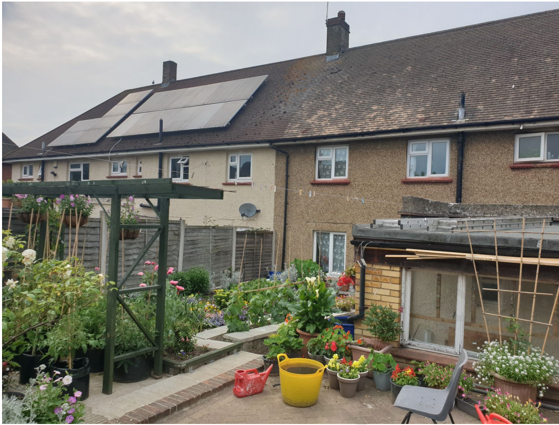
FIGURE 5: Dwelling houses at 6 & 8 Dorchester Road.
