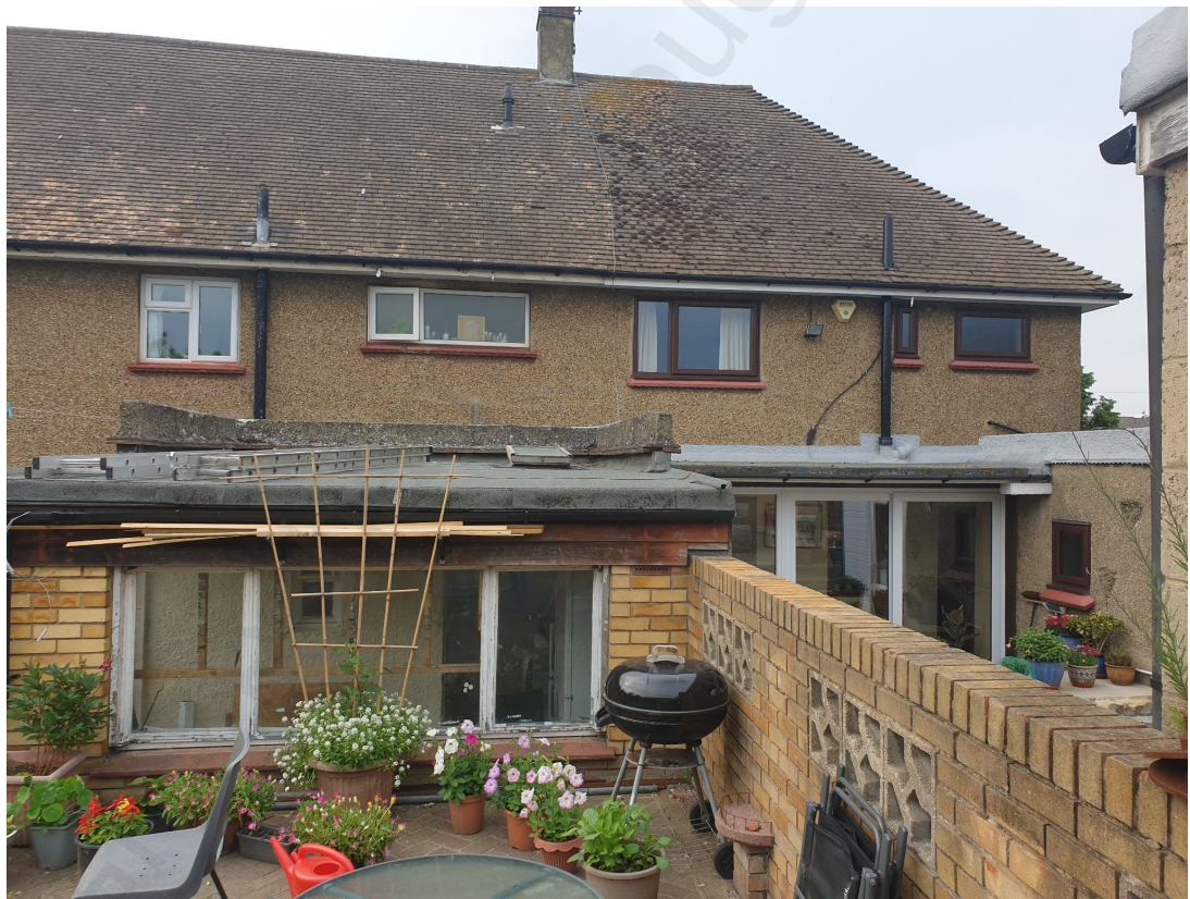
FIGURE 4: Dwelling houses at 8 & 10 Dorchester Road.
