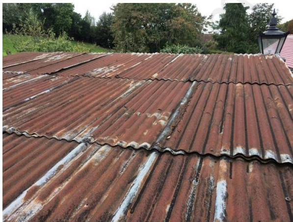
Figure 3: Previous metal sheet roofing
