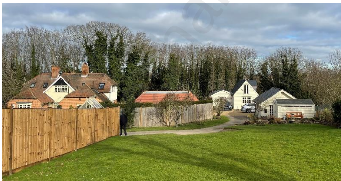
Figure 5: Outbuilding within its setting
