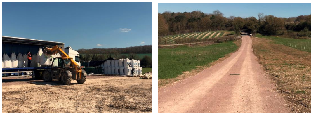
Compost being delivered to the site along access track
