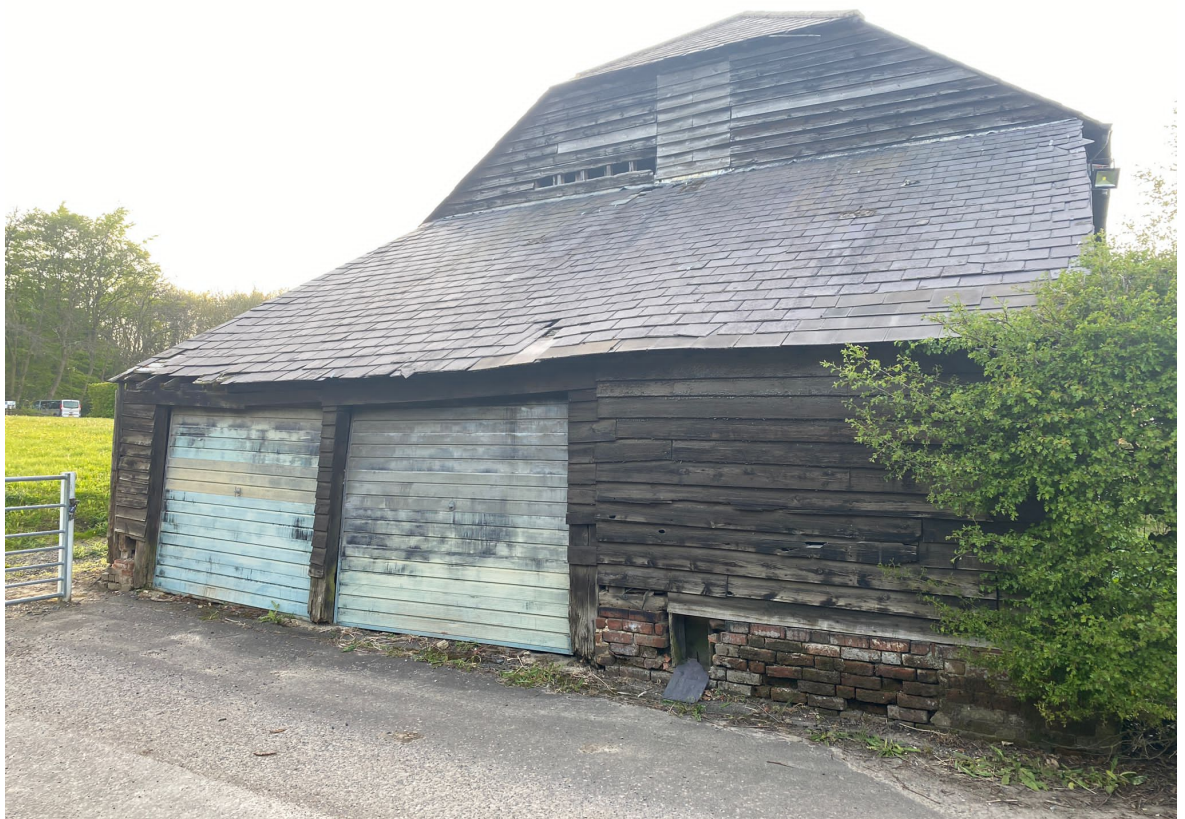
Photograph 1. Parsonage Farm Barn
