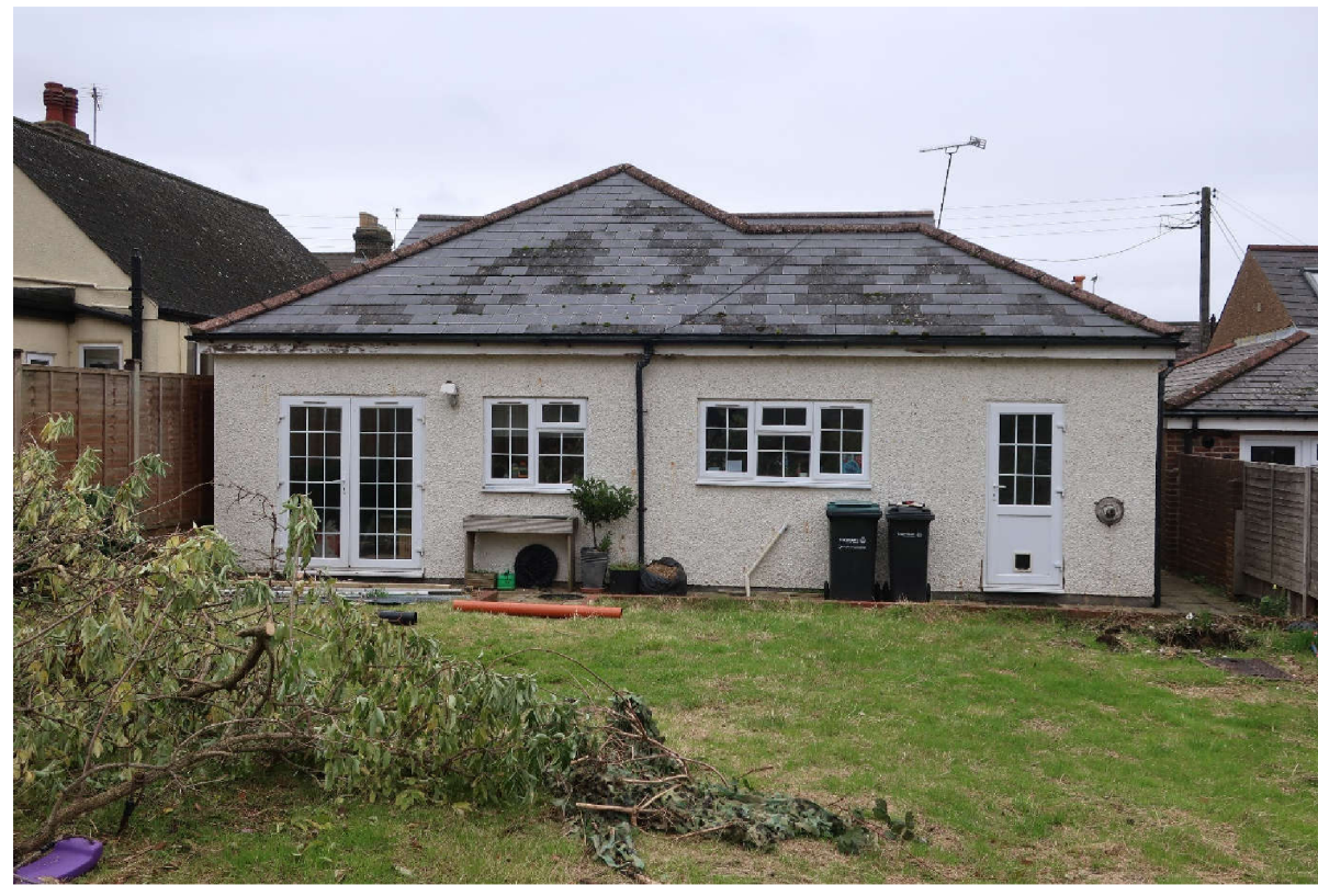
Photo 2 Looking at the Rear of No 5 Forge Lane
