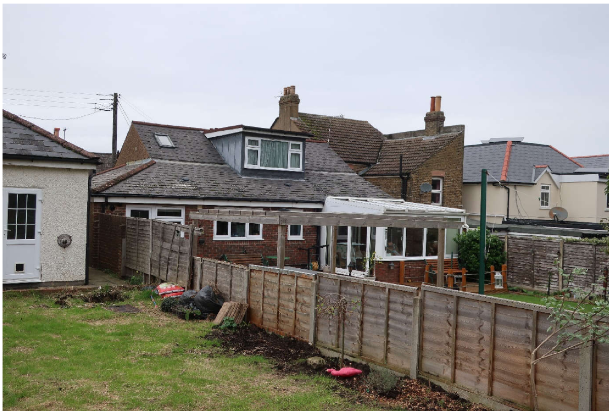
Photo 3 Looking northwards – Flat roof to Commercial property.
