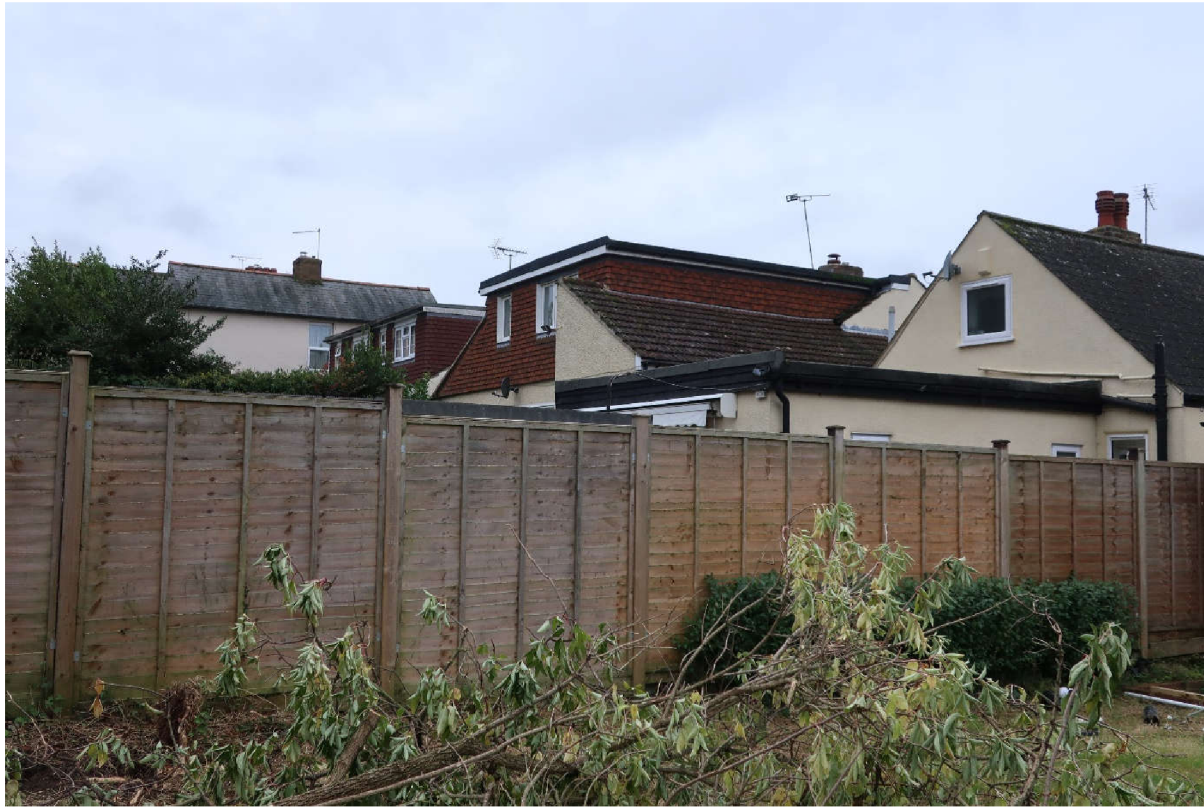
Photo 1 Property to the South
