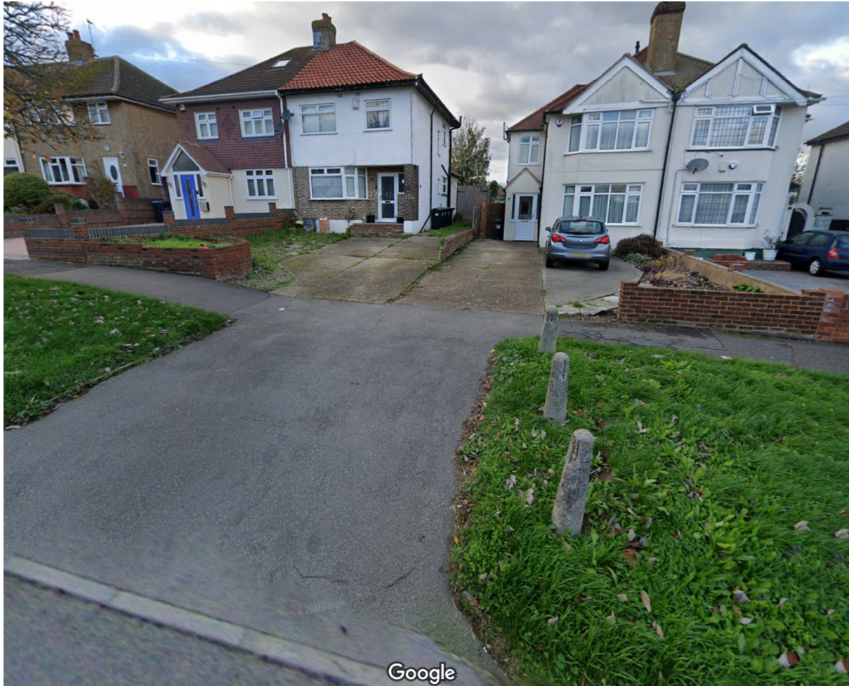
Double crossover and dropped kerb found at No. 34 and 36 Thong Lane.
