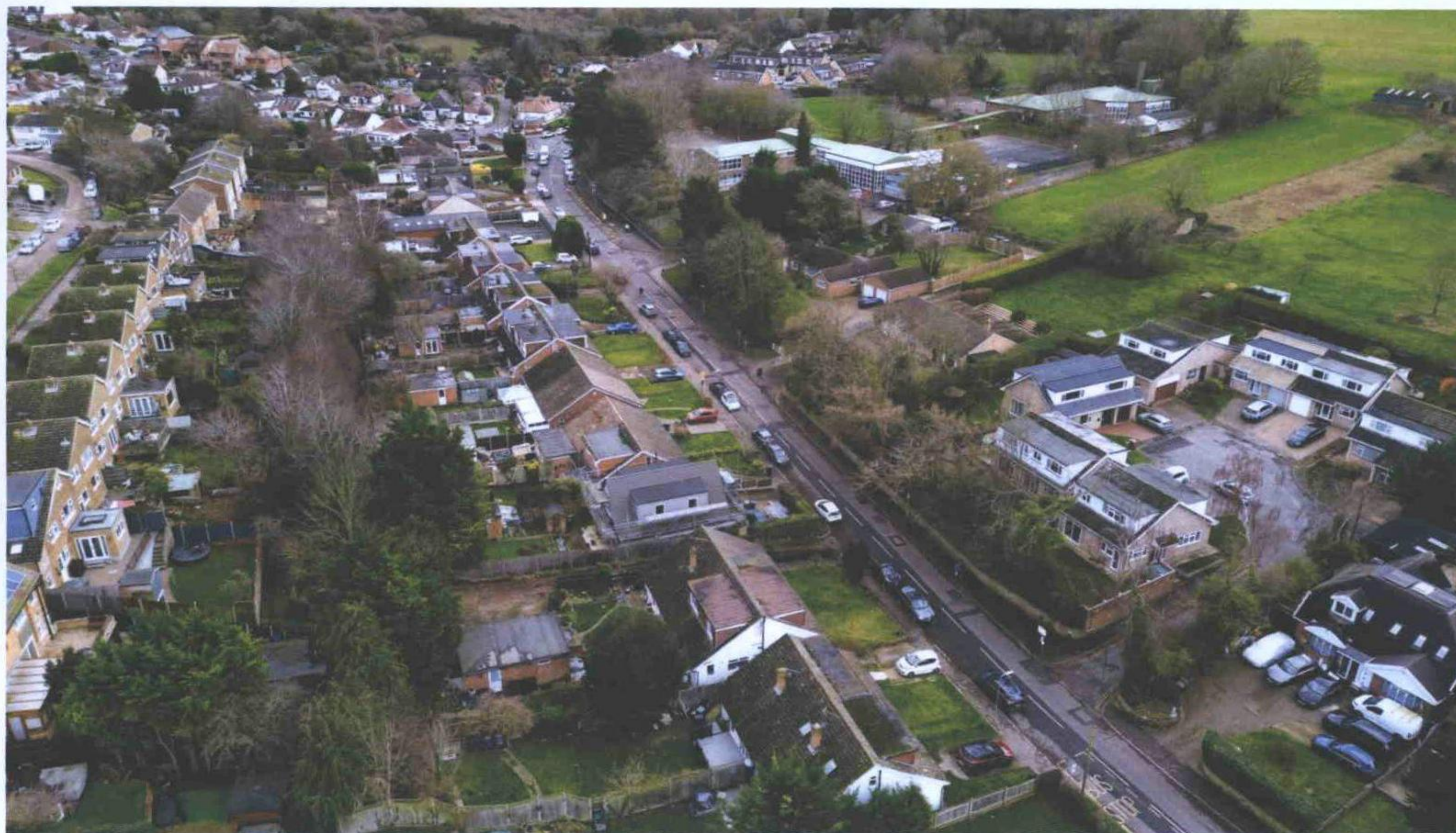
Another view of part of the site from above Downs Road looking towards the school.
